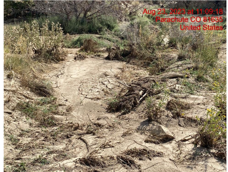
Degradation of Access Road/Insufficient Erosion Control – Photo #06087
