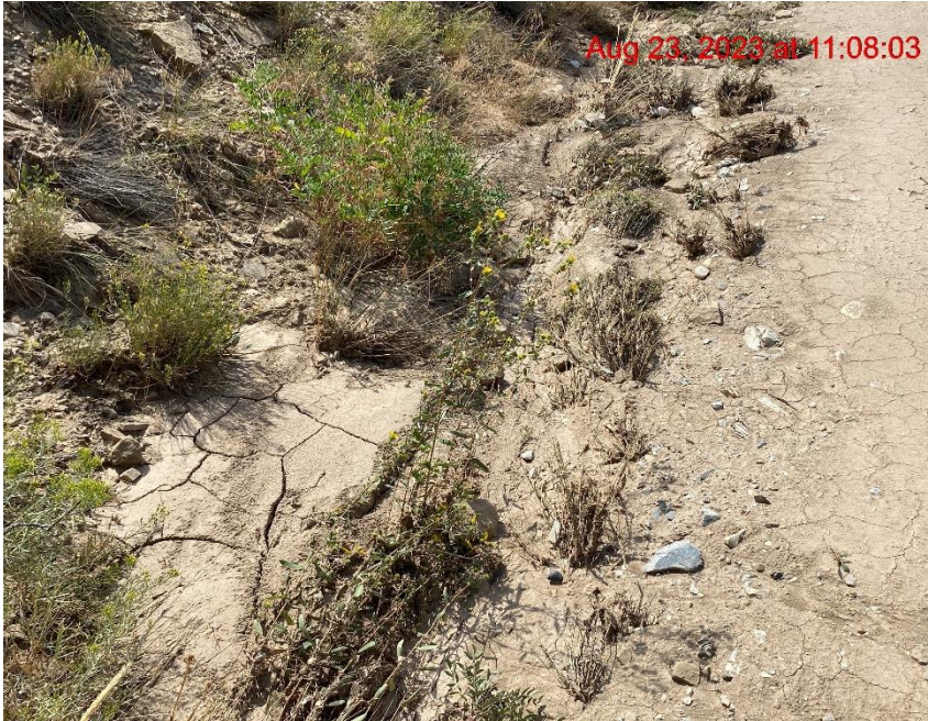
Degradation of Access Road/Insufficient Erosion Control – Photo #06084
