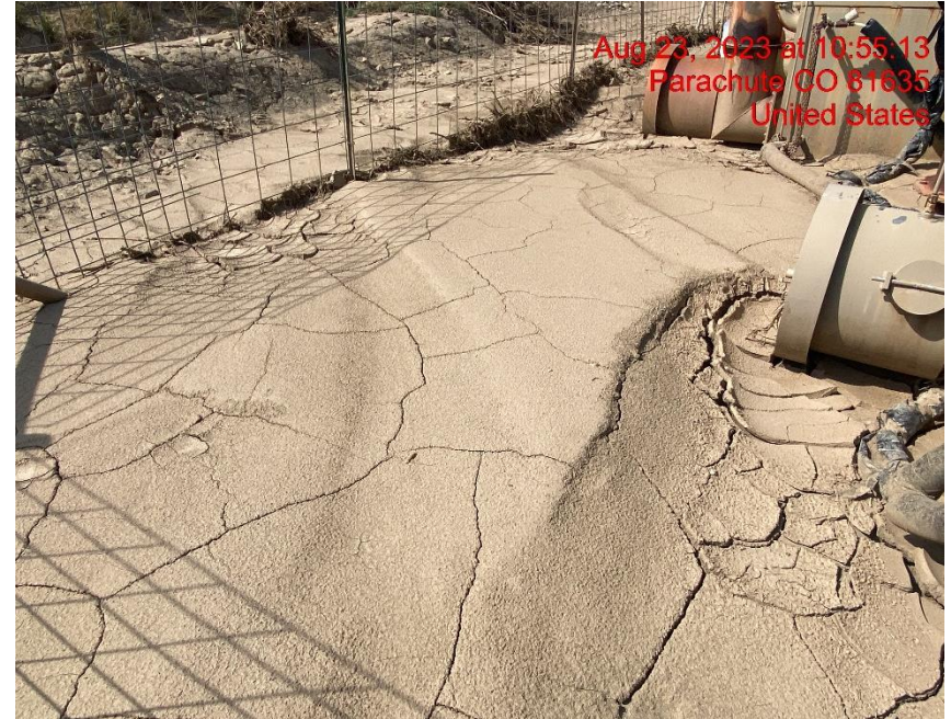
Insufficient Erosion Control/Sediment Run-On to Location – Photo #06079
