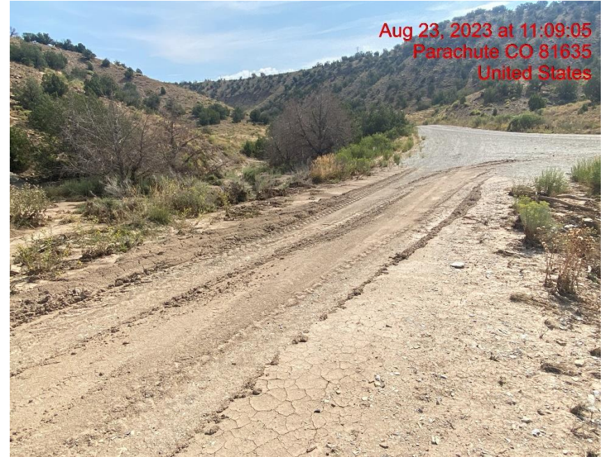
Insufficient Vehicle Tracking BMPs at Location Entrance/Exit – Photo #06086
