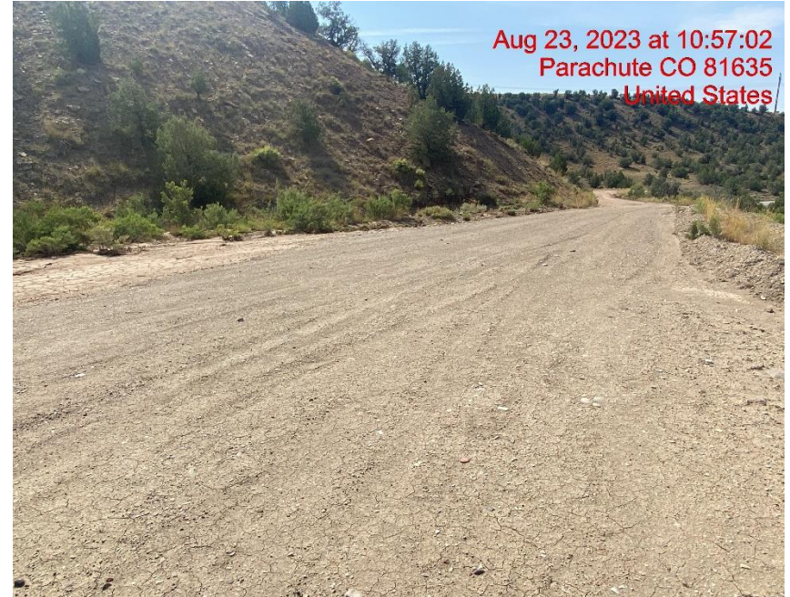
Insufficient Vehicle Tracking BMPs at Location Entrance/Exit – Photo #06081
