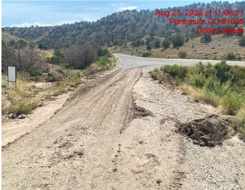
Degradation of Access Road/Insufficient Erosion Control – Photo #06085
