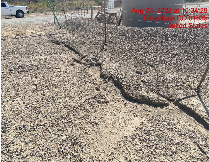
Insufficient Erosion Control Near Tank Battery – Photo #06066
