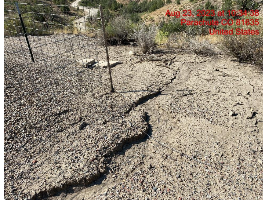
Insufficient Erosion Control Near Tank Battery – Photo #06067
