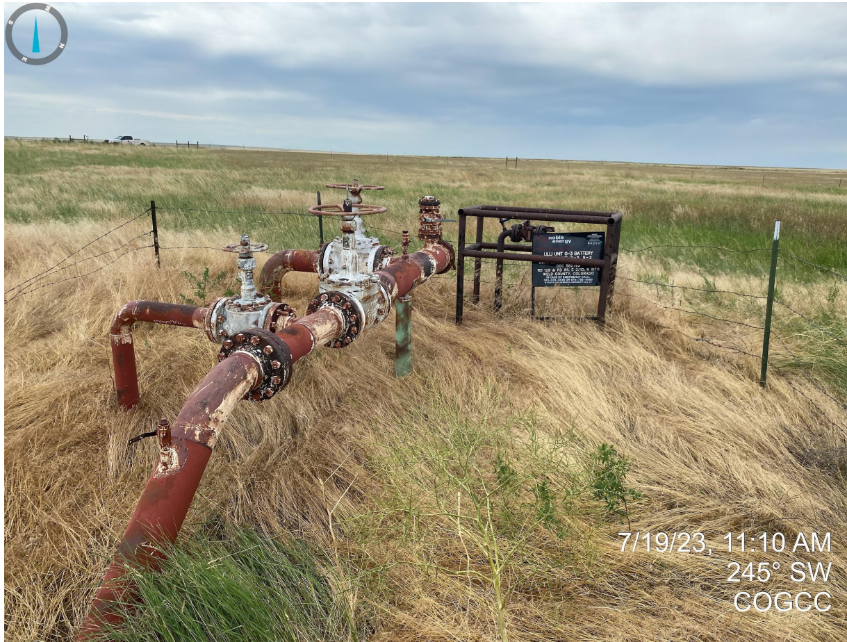
Photo 5. Pipe risers remain on location; this equipment was documented in previous inspections (dating back to 07/31/2017; Doc #675103782) and has yet to be removed. All equipment must be removed from the abandoned location.
