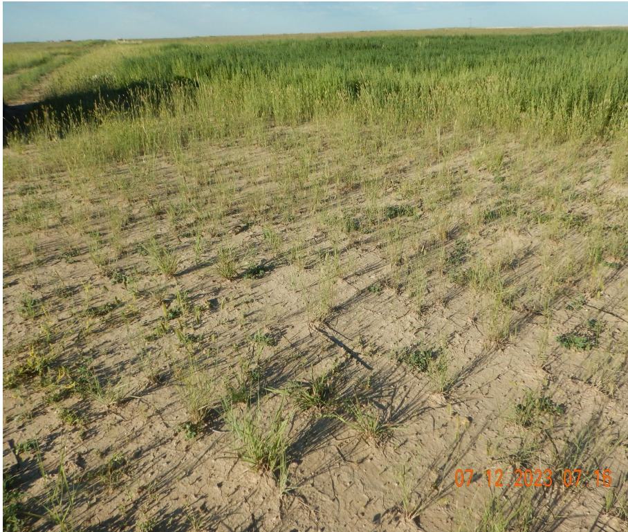
Photo 4. Photo taken from an area of the excavation, facing South. Photo illustrates the excavation area was seeded but with introduced species that is not reflective of reference area species.
