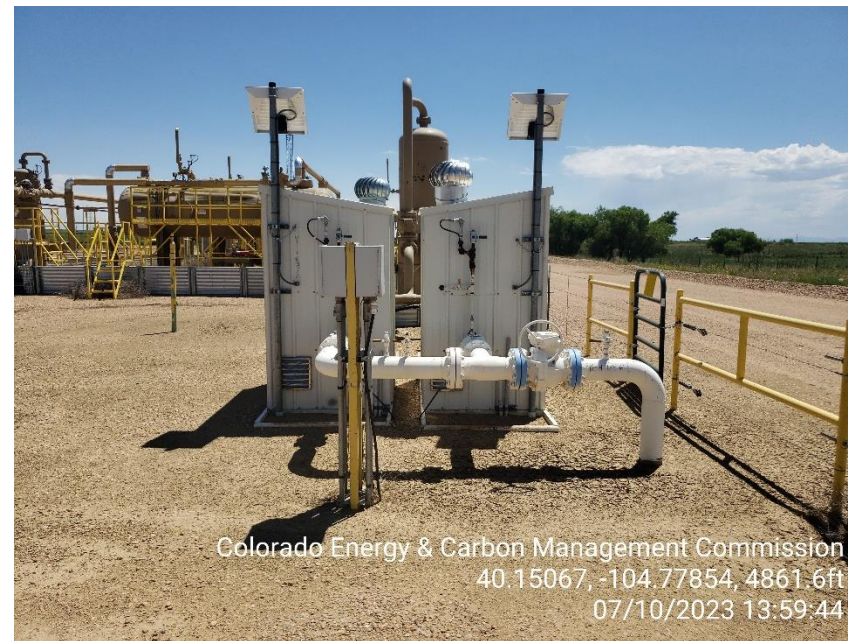
Photo 12 Gas Meter Runs.
