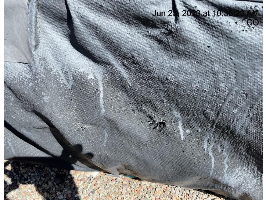
Photo # 1636 Hole in containment liner/liner needs maintenance
