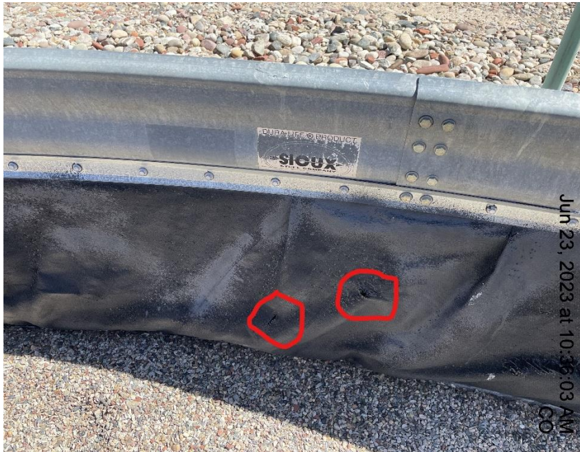
Photo # 1631 Holes in containment liner/liner needs maintenance
