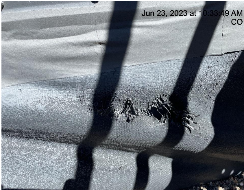
Photo # 1617 Hole in containment liner/liner needs maintenance
