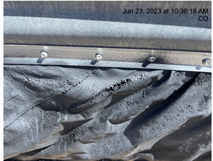
Photo # 1634 Hole in containment liner/liner needs maintenance
