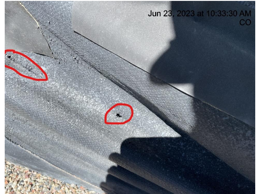
Photo # 1614 Holes in containment liner/liner needs maintenance
