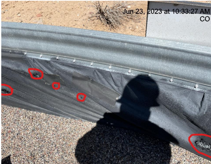
Photo # 1613 Holes in containment liner/liner needs maintenance
