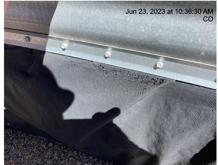
Photo # 1638 Holes in containment liner/liner needs maintenance
