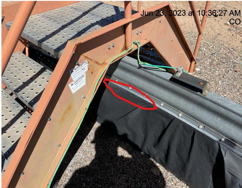
Photo # 1637 Holes in containment liner/liner needs maintenance
