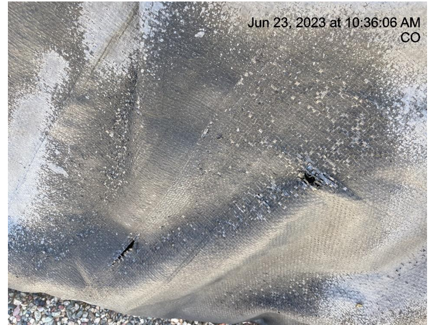
Photo # 1632 Holes in containment liner/liner needs maintenance
