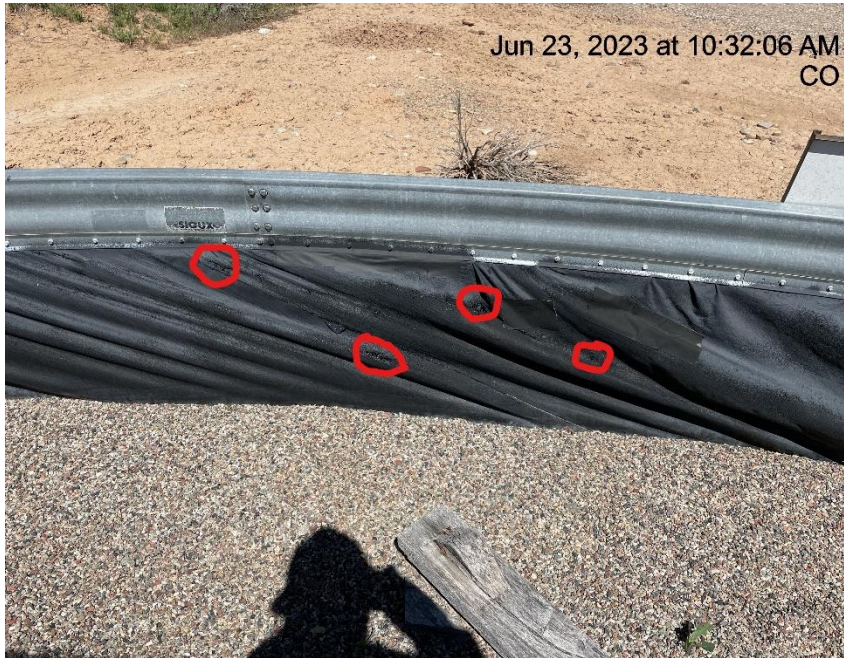
Photo # 1609 Holes in containment liner/liner needs maintenance
