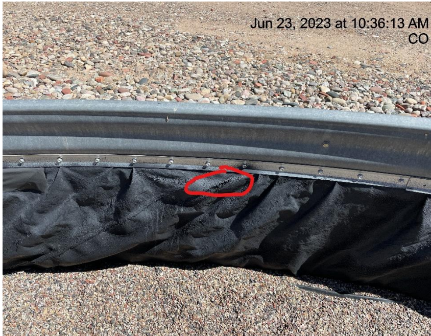
Photo # 1633 Hole in containment liner/liner needs maintenance
