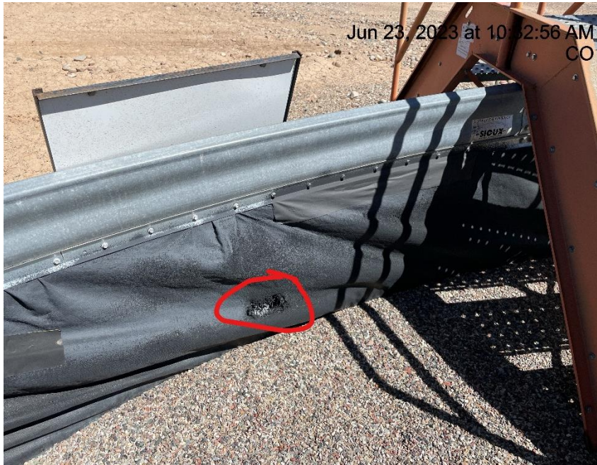
Photo # 1611 Hole in containment liner/liner needs maintenance
