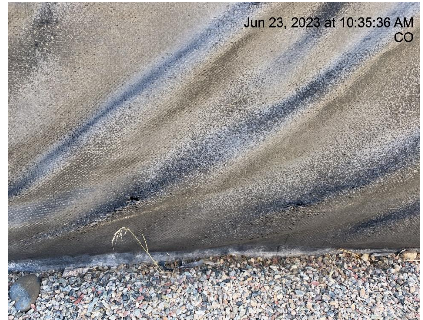
Photo # 1628 Holes in containment liner/liner needs maintenance
