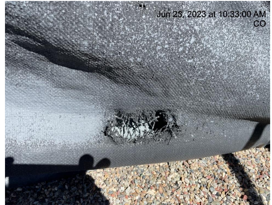
Photo # 1612 Hole in containment liner/liner needs maintenance
