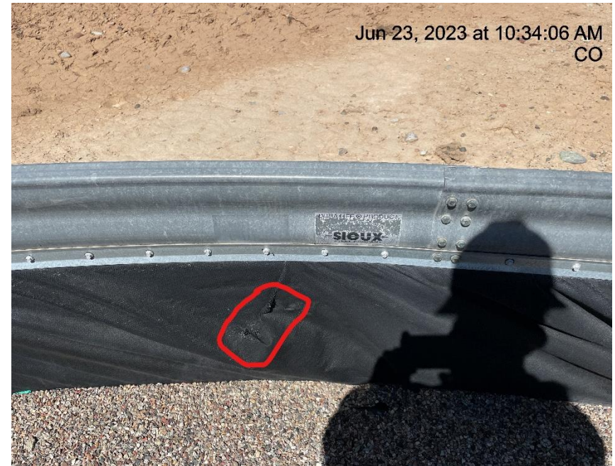
Photo # 1620 Holes in containment liner/liner needs maintenance
