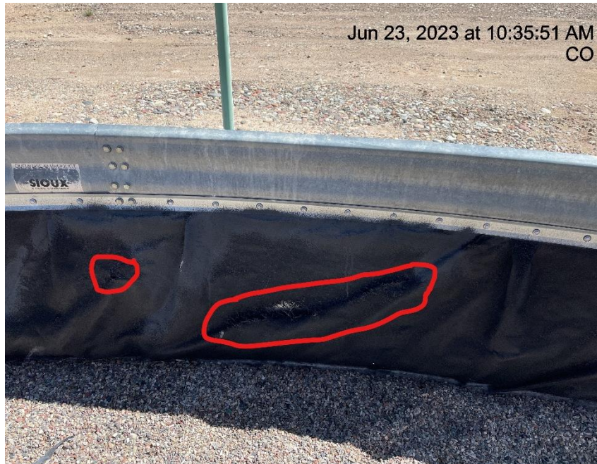
Photo # 1629 Holes in containment liner/liner needs maintenance
