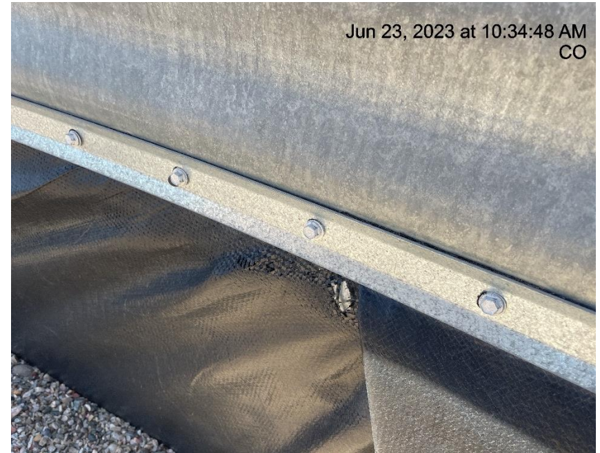
Photo # 1626 Hole in containment liner/liner needs maintenance
