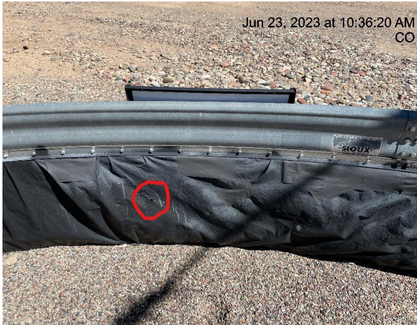
Photo # 1635 Hole in containment liner/liner needs maintenance
