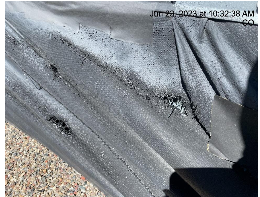
Photo # 1610 Holes in containment liner/liner needs maintenance
