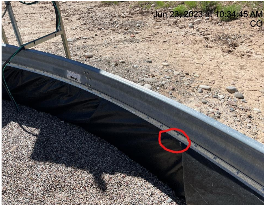
Photo # 1625 Hole in containment liner/liner needs maintenance
