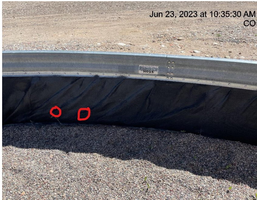
Photo # 1627 Holes in containment liner/liner needs maintenance
