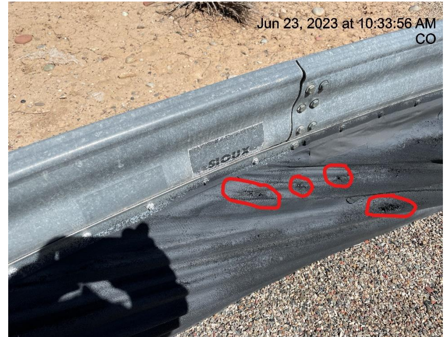
Photo # 1618 Holes in containment liner/liner needs maintenance
