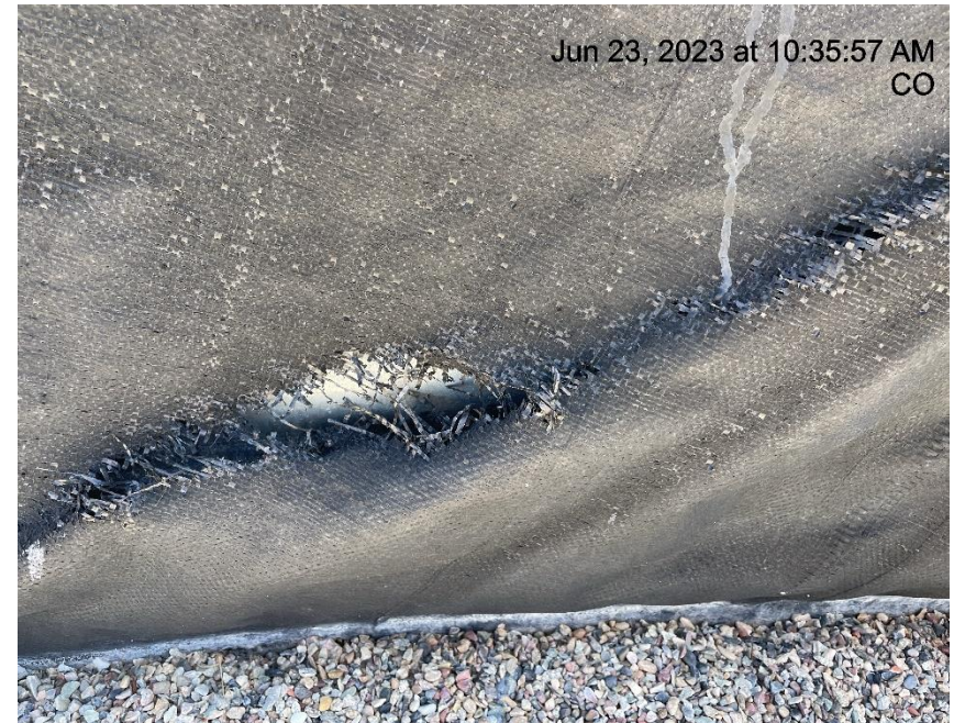
Photo # 1630 Holes in containment liner/liner needs maintenance
