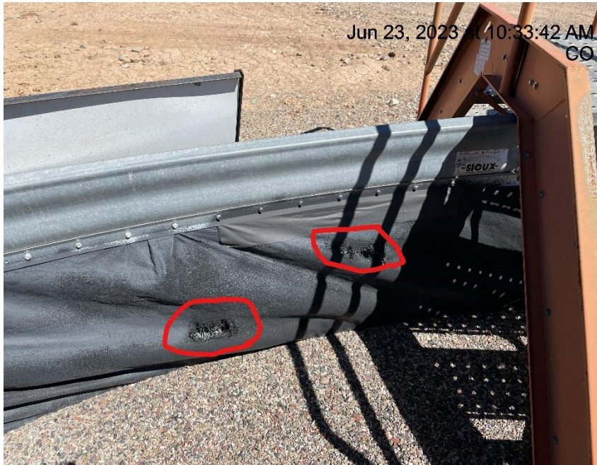
Photo # 1615 Holes in containment liner/liner needs maintenance
