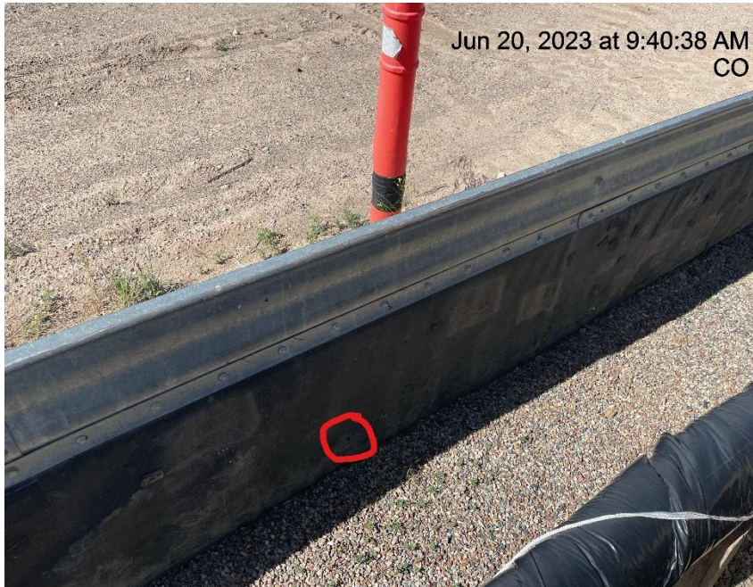
Photo # 1078 Hole in liner/liner needs maintenance
