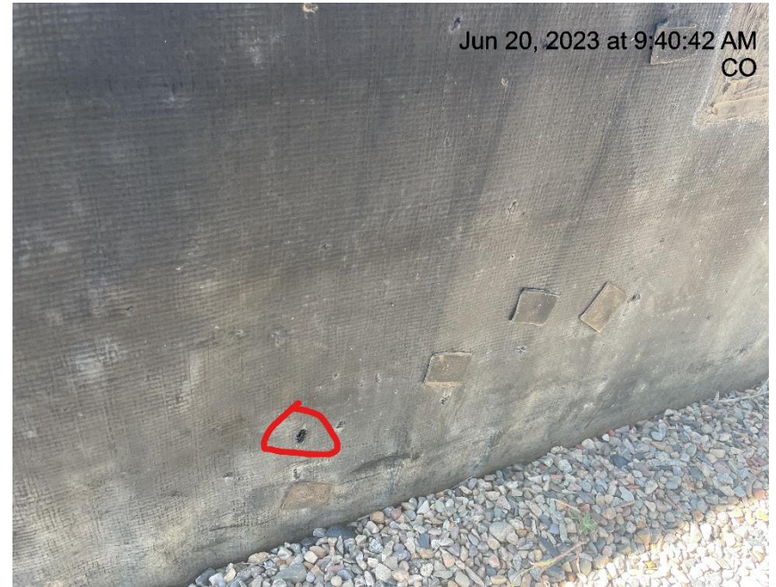
Photo # 1079 Hole in liner/liner needs maintenance
