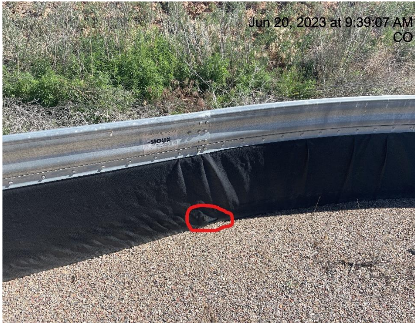
Photo # 1072 Hole in liner/liner needs maintenance
