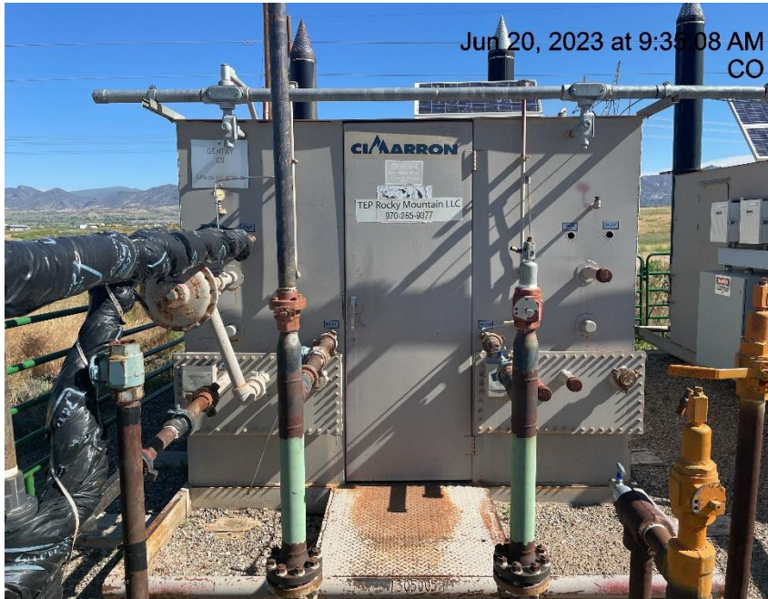
Photo # 1067 Meter calibration info not conspicuously posted
