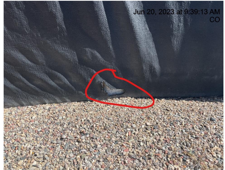
Photo # 1073 Hole in liner/liner needs maintenance
