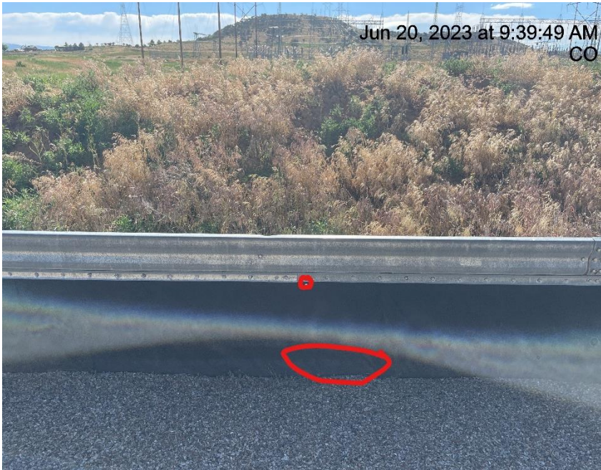
Photo # 1074 Holes in liner/liner needs maintenance
