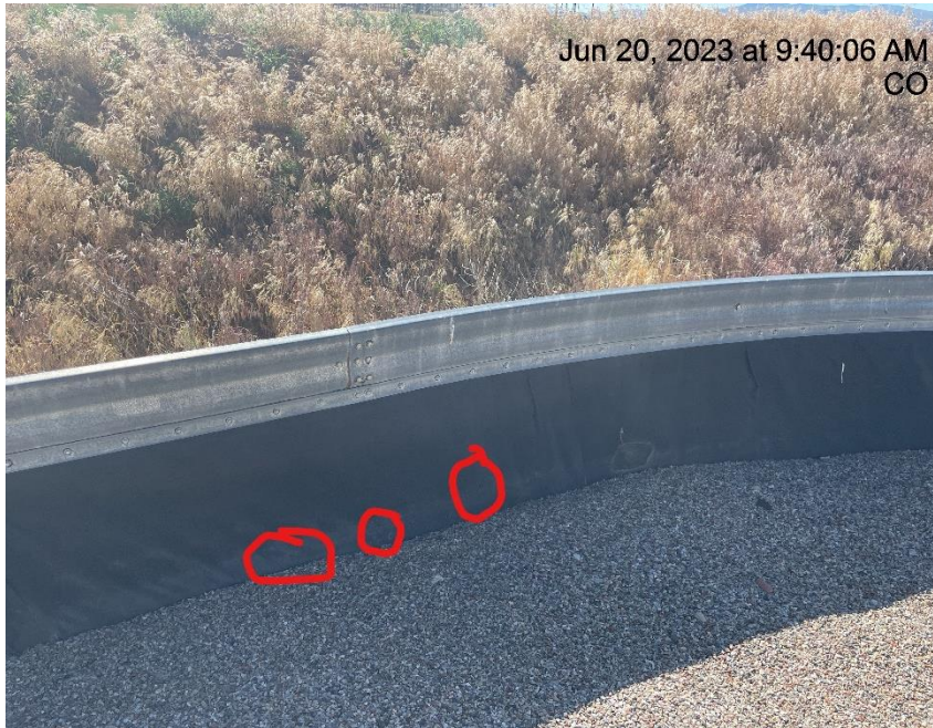
Photo # 1076 Holes in liner/liner needs maintenance
