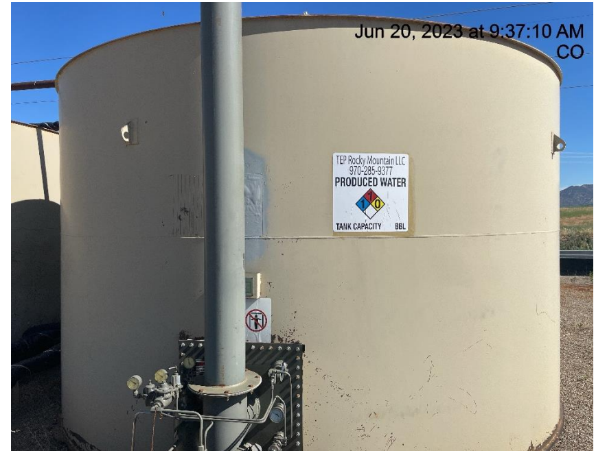
Photo # 1071 Tank label missing required information
