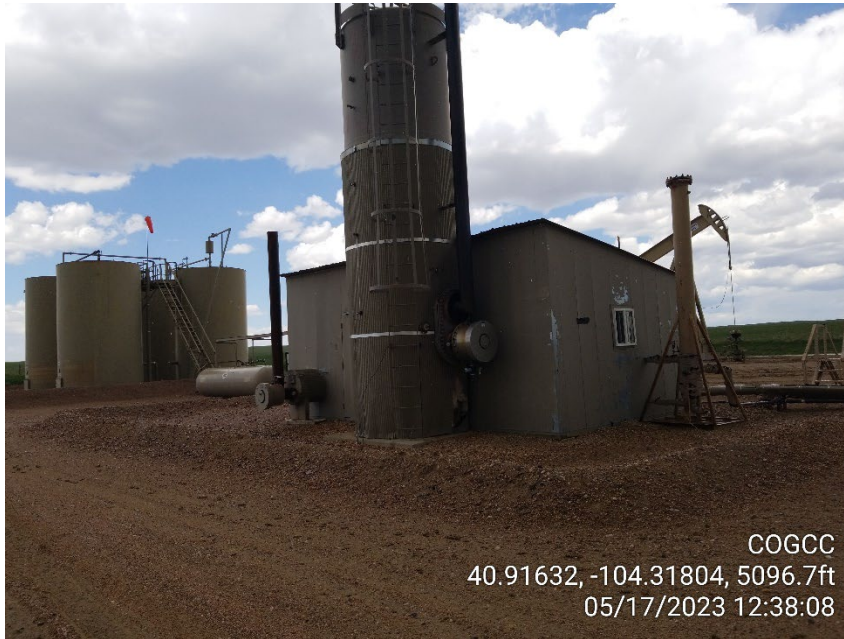
Photo 3 – Heater Treater
