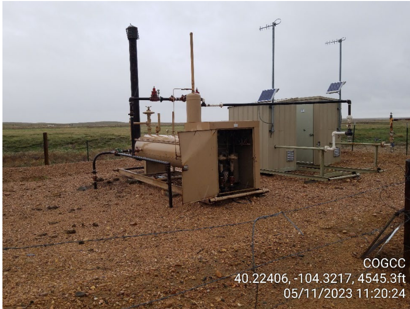
Photo 5 – Separator and Gas Meters
