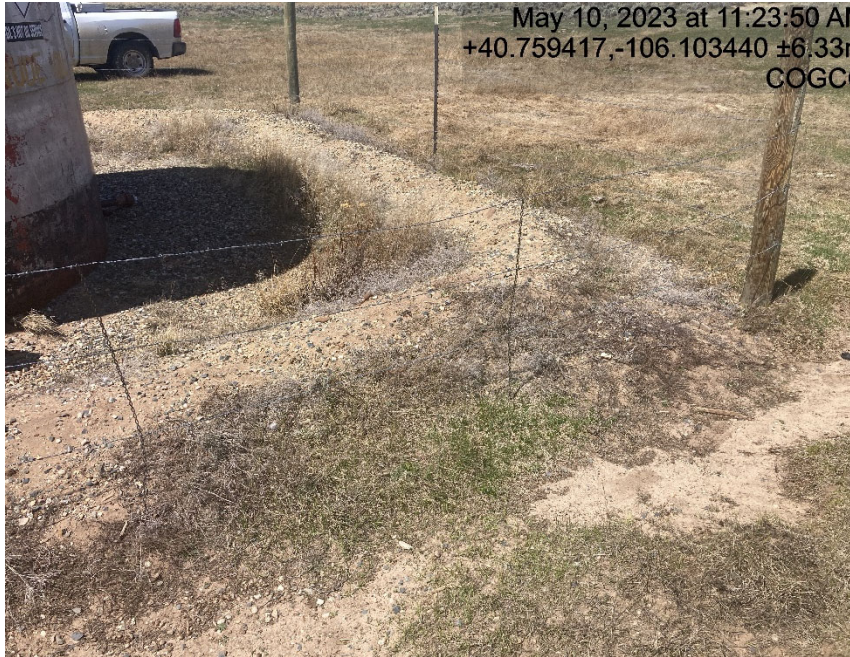
Insufficient secondary containment and weeds
