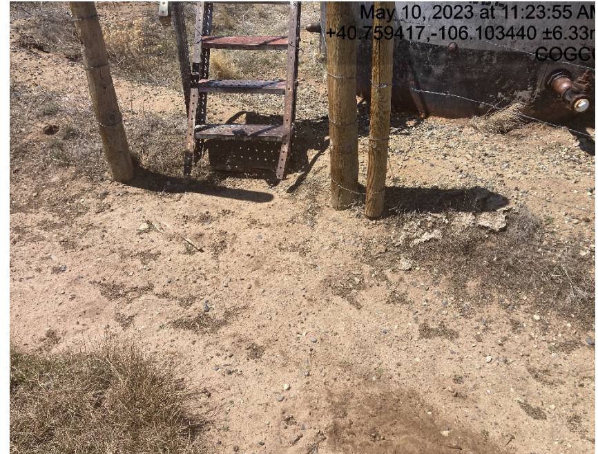
Insufficient secondary containment and weeds
