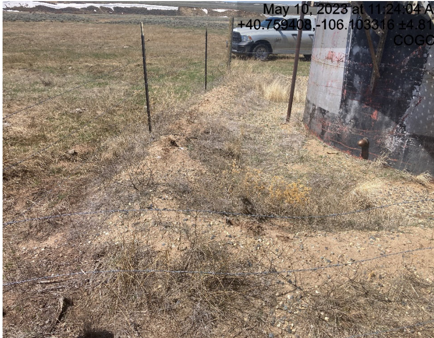
Insufficient secondary containment and weeds
