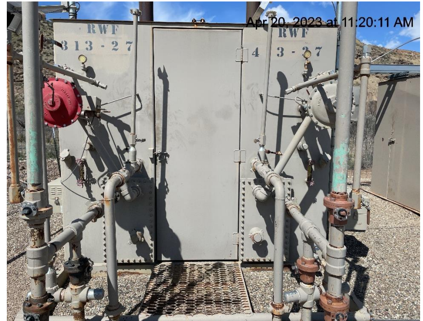
Photo # 5952 Meter calibration info not conspicuously posted
