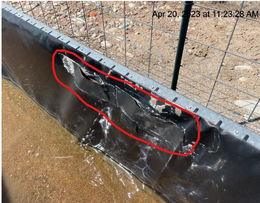
Photo # 5955 Containment liner needs maintenance
