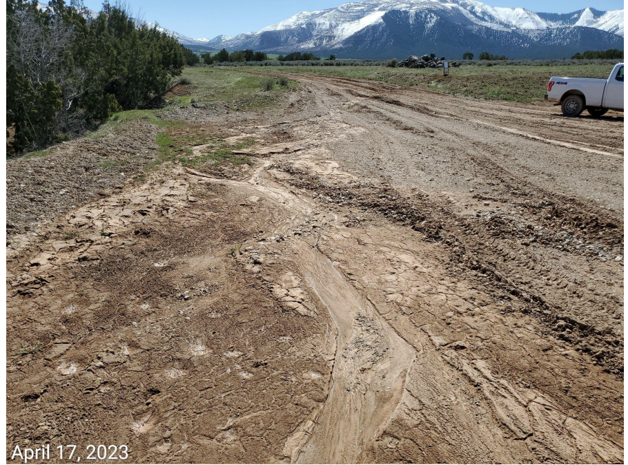
Photo 3: Pad lacks stabilization. Stormwater and erosion controls missing or insufficient.
