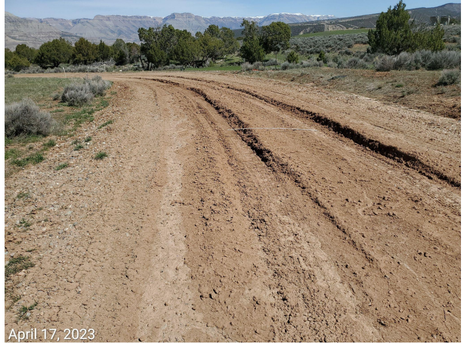
Photo 11: Photos examples showing stormwater and erosion control BMPs along access road are missing or insufficient. 6 foot measuring stick for reference.
