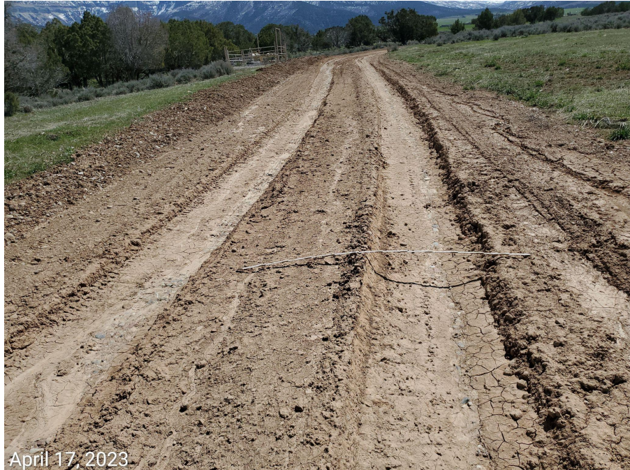
Photo 11: Photos examples showing stormwater and erosion control BMPs along access road are missing or insufficient. 6 foot measuring stick for reference.
