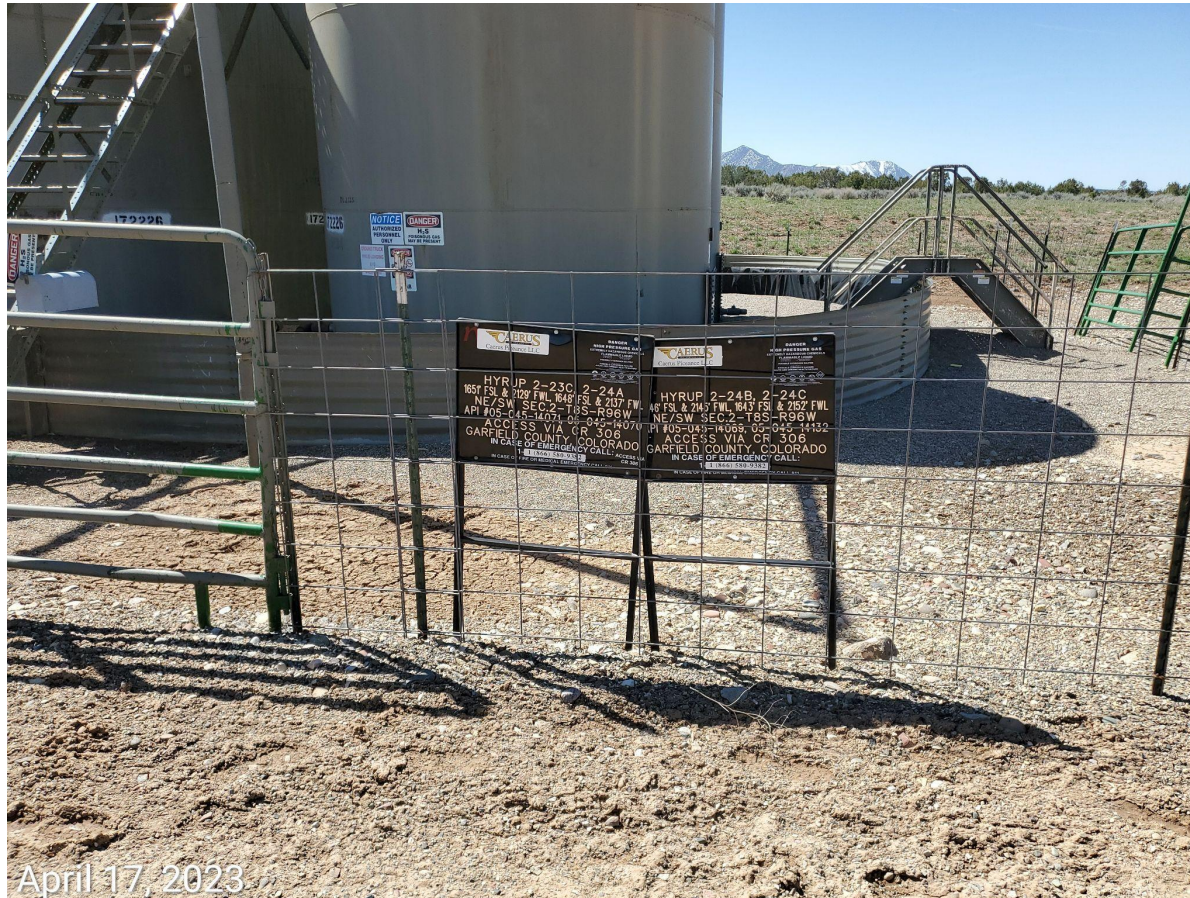
Photo 5: Tank battery signage. Photo also show signs or labels at tanks not posted or information too small to read at distance or installed in place where not visible.
