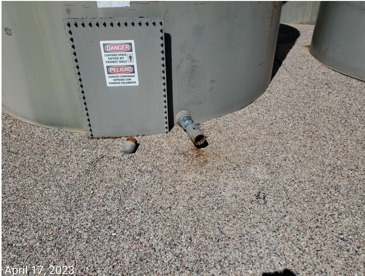
Photo 7: Plug removed from tank. Small leak appears evident. Plug requires replacement and impacted materials removed.
