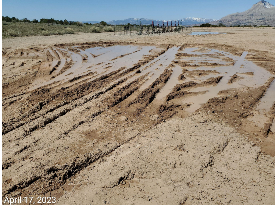
Photo 3: Pad lacks stabilization. Stormwater and erosion controls missing or insufficient.
