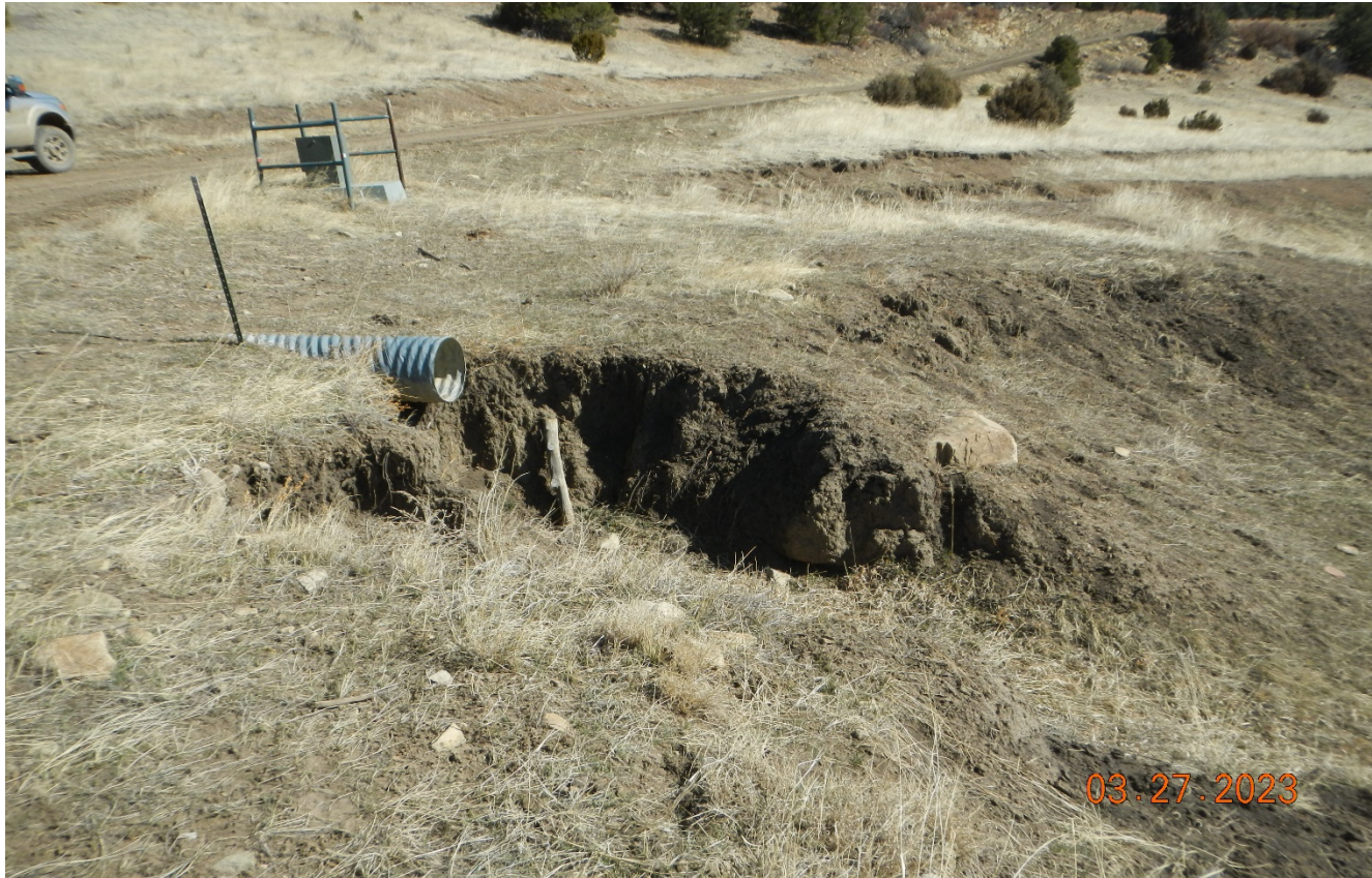
Photo 3. Facing northeast at the same area of the road as previous photos. This culvert outlet has eroded and needs to be repaired along with outlet protection.
