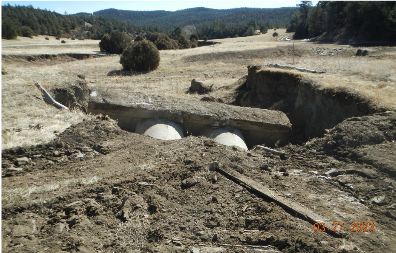
Photo 2. Facing east at the same point in the road as previous photo. There is a cement culvert pushed into the erosion embankment which needs to be removed and the embankment needs to be stabilized.
