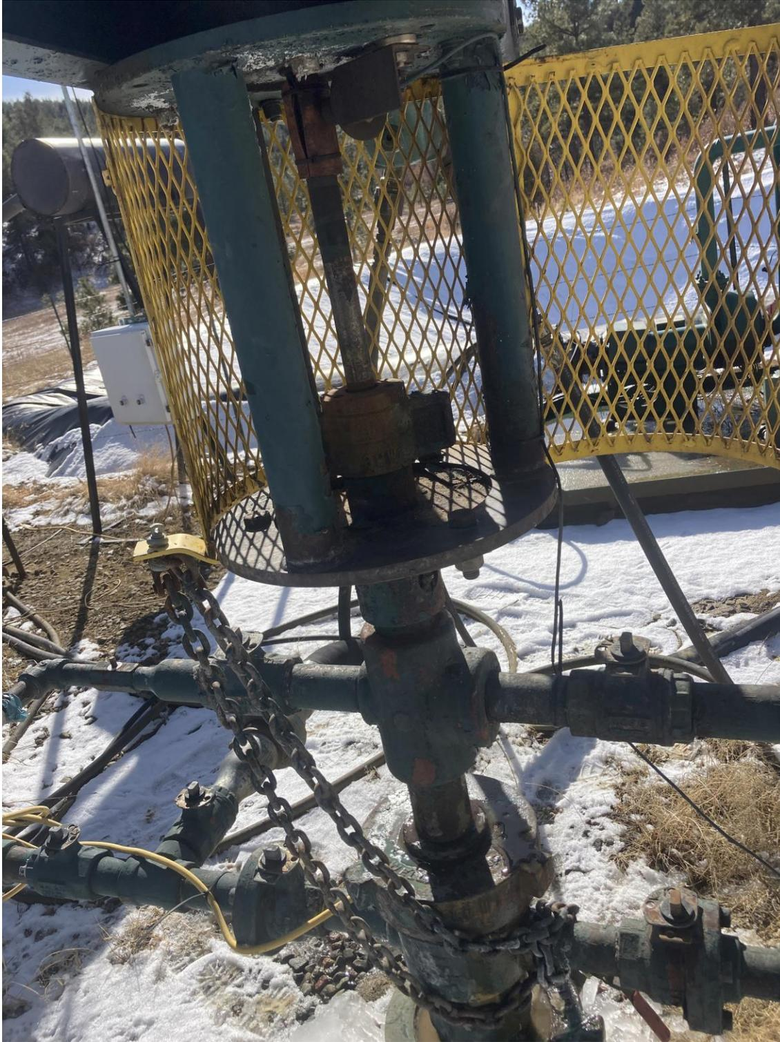
Controlled and contained spill release and cleaned per Rule 912. Securely fastened all valves, pipes, and fitting to ensure good mechanical condition, will inspected on regular intervals and maintain in good mechanical condition per Rule 608.
