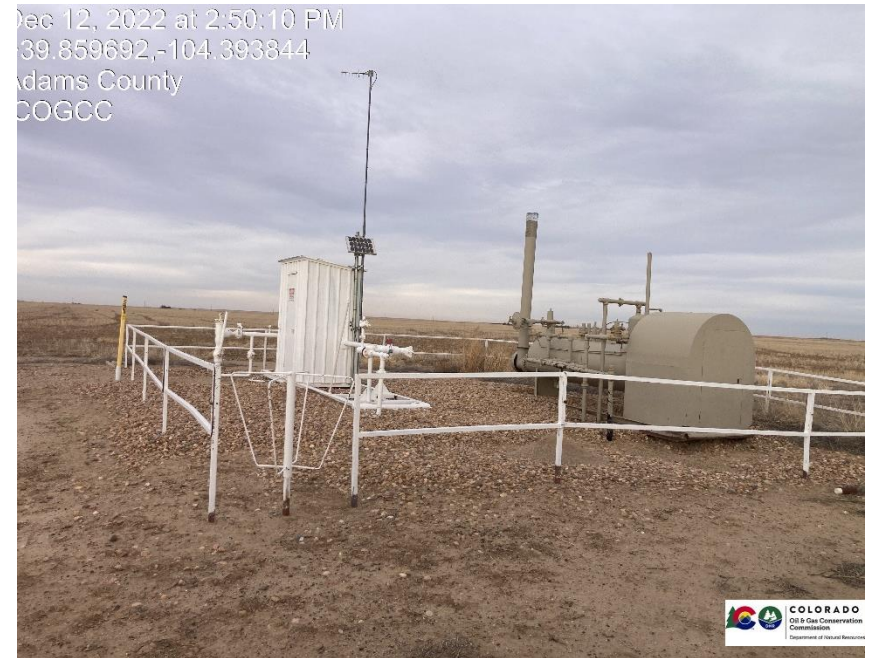
Pic 4 Separator, Gas meter run.
