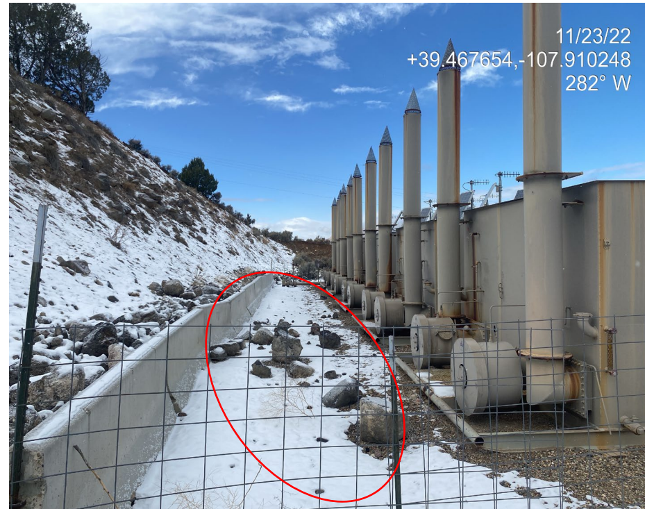
Photo 11. Photo from 11/23/22 inspection shows additional rocks have fallen over the jersey barrier from the cut slope indicating continued erosion of slopes.
