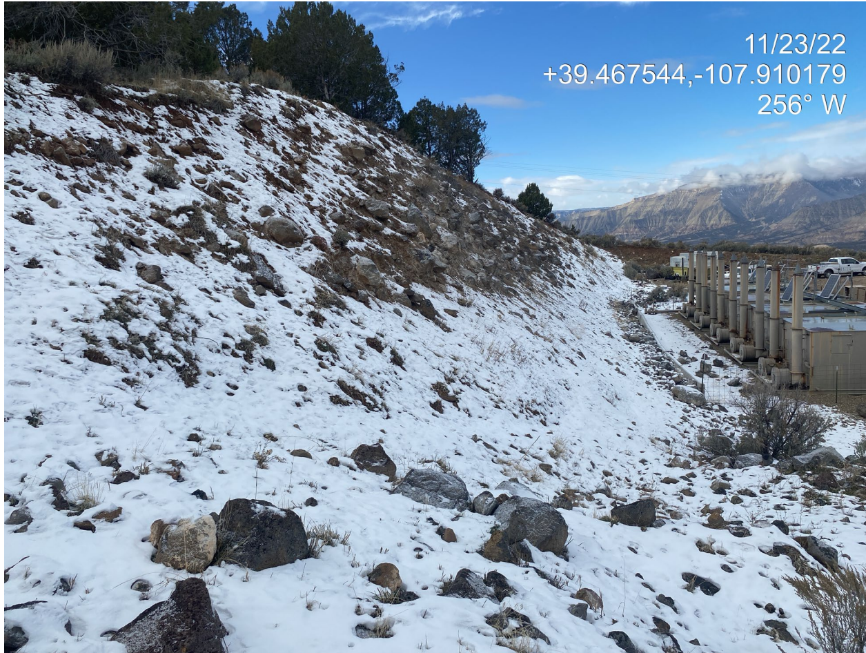
Photo 9. Photo shows the cut slope to the south of the location behind the separators. Note rocks fallen within separator area past jersey barrier.
