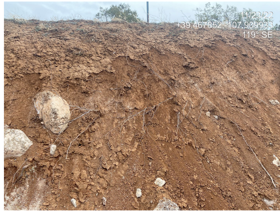
Photo 8. Photo shows a close-up of the eroding cut slope at the east of the location. Note exposed roots indicating soil loss.
