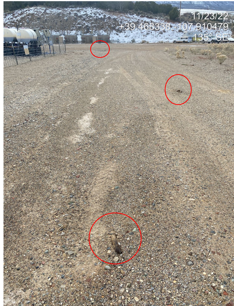
Photo 3. Photo shows unmarked anchors to the west of the wells.
