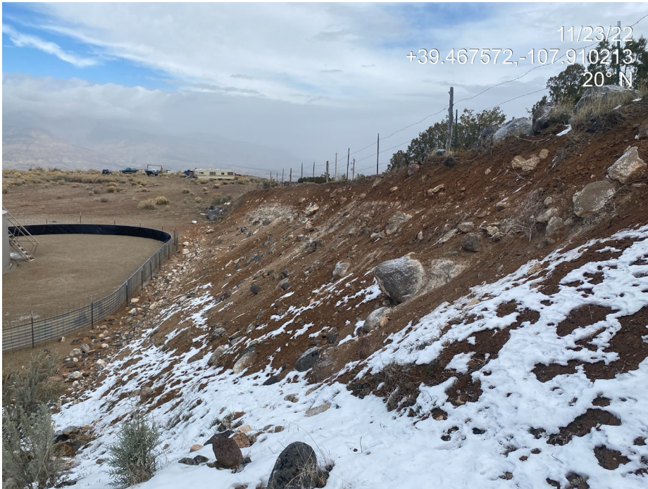
Photo 7. Photo shows an overview of the eroding cut slope at the east of the location.
