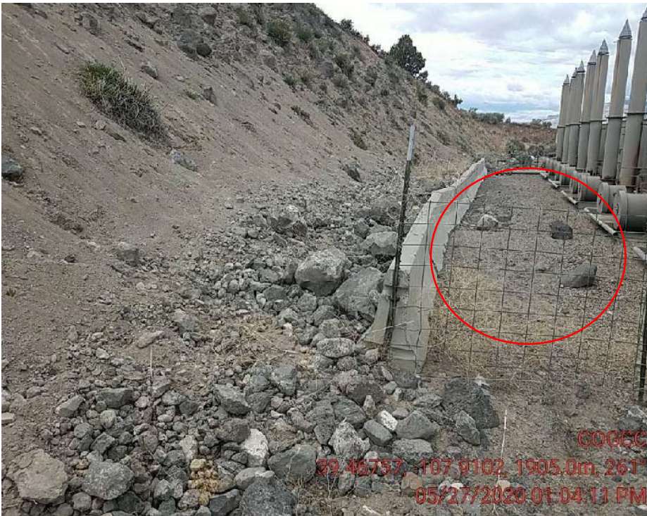
Photo 10. Photo taken 5/27/2022 from inspection #700700789 shows approximately three rocks have fallen over the jersey barrier from the cut slope.
