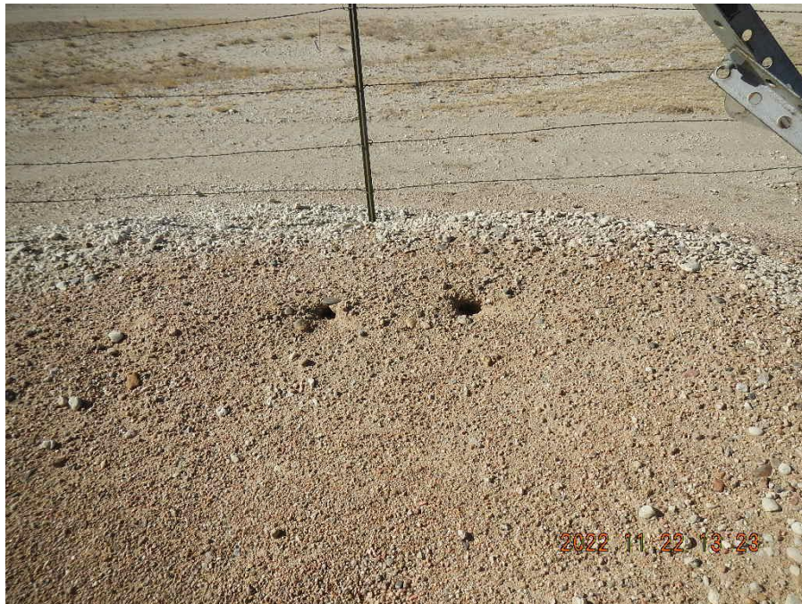
Photo 9. Burrows compromising secondary containment berm.
