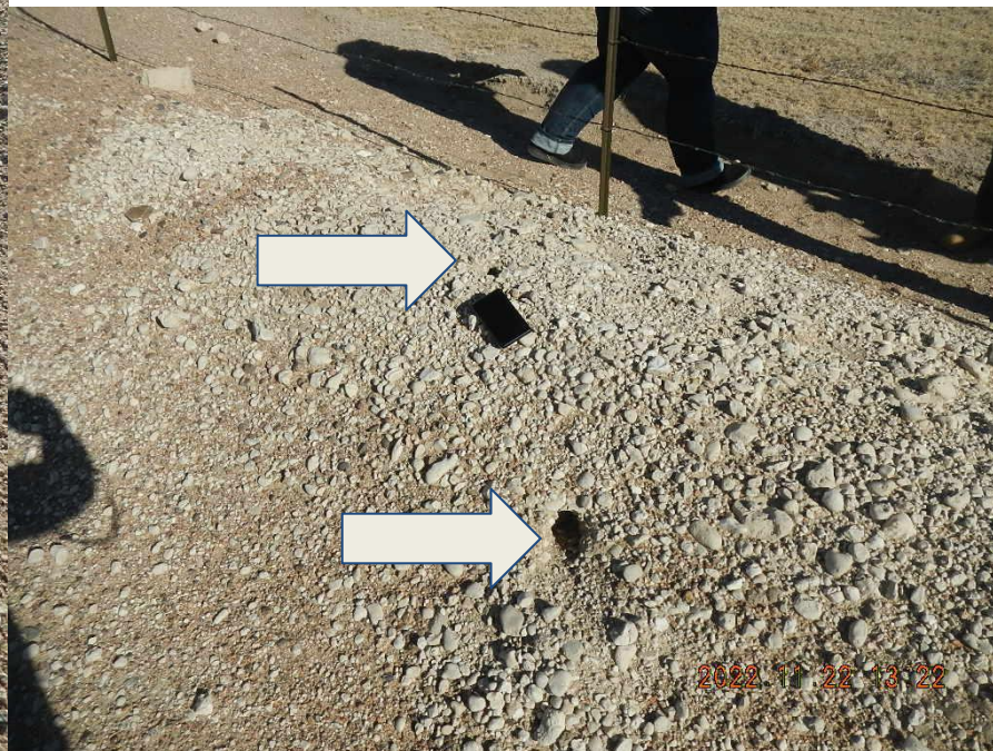
Photo 8. Burrows compromising secondary containment berm.
