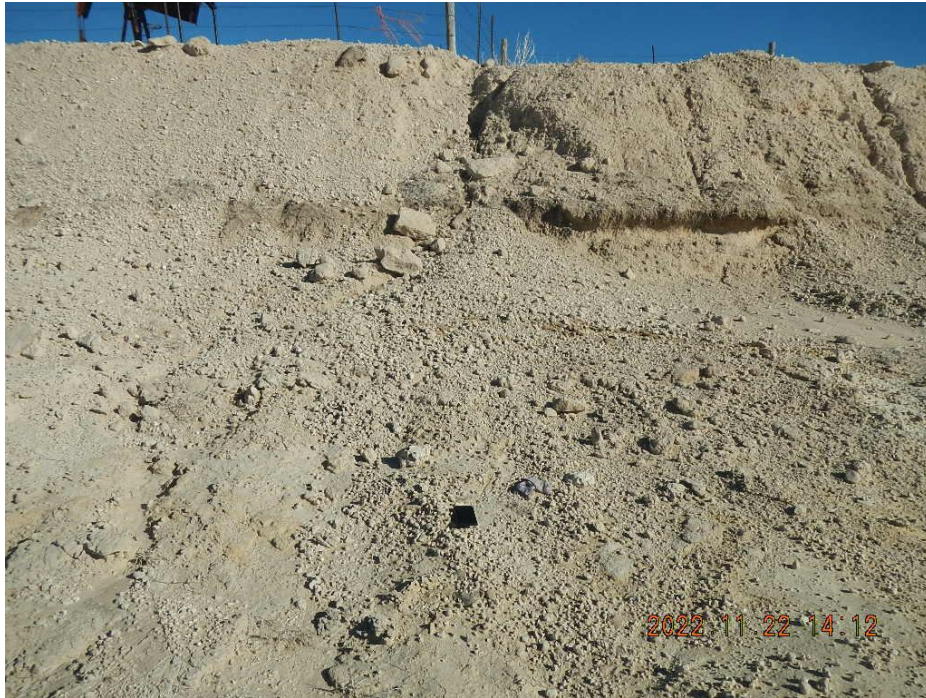
Photo 25. Signs of stormwater run on into the pit.
