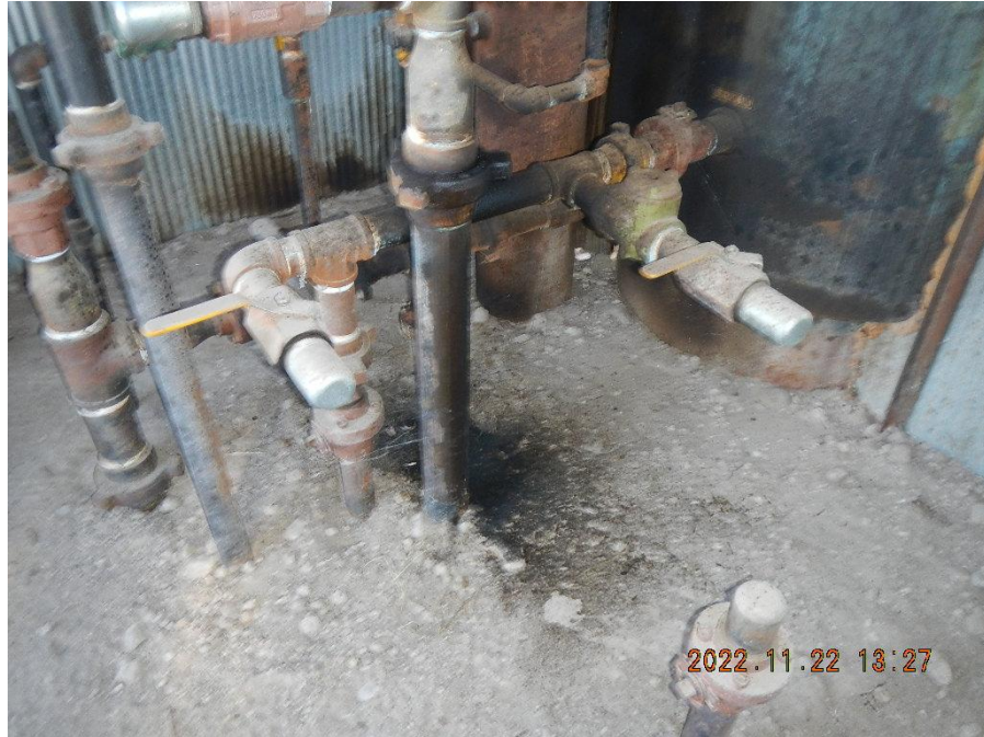
Photo 11. Hammer union weeping oil and oil staining on ground.
