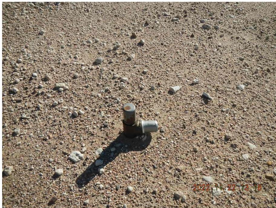
Photo 7. Un-marked riser at tank battery.
