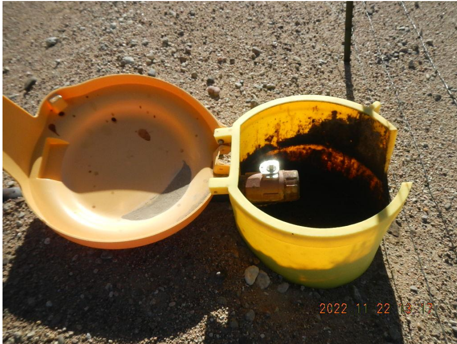
Photo 3. Loadout containment basin found open.
