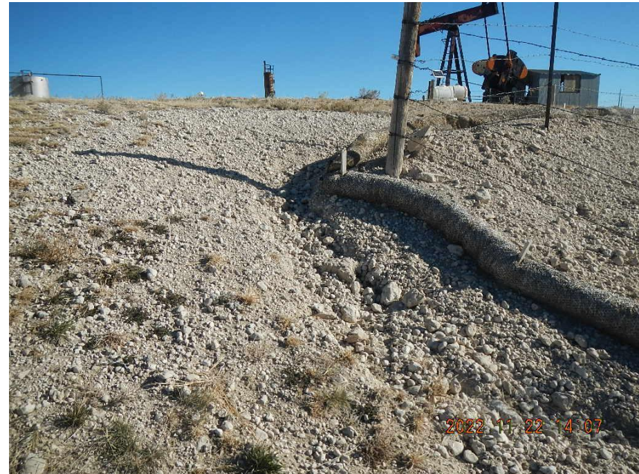
Photo 30. Erosion along the north side of the pit.
