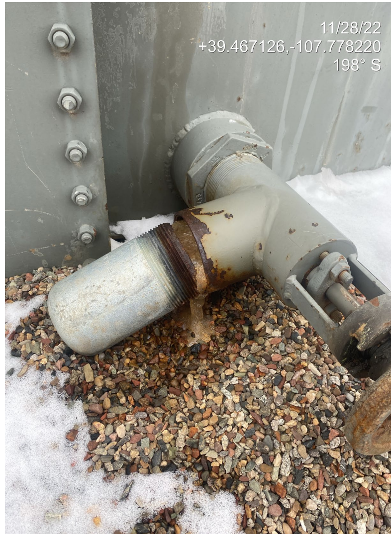
Photo 2. Photo shows fluid leaking from a produced water/condensate tank drain.
