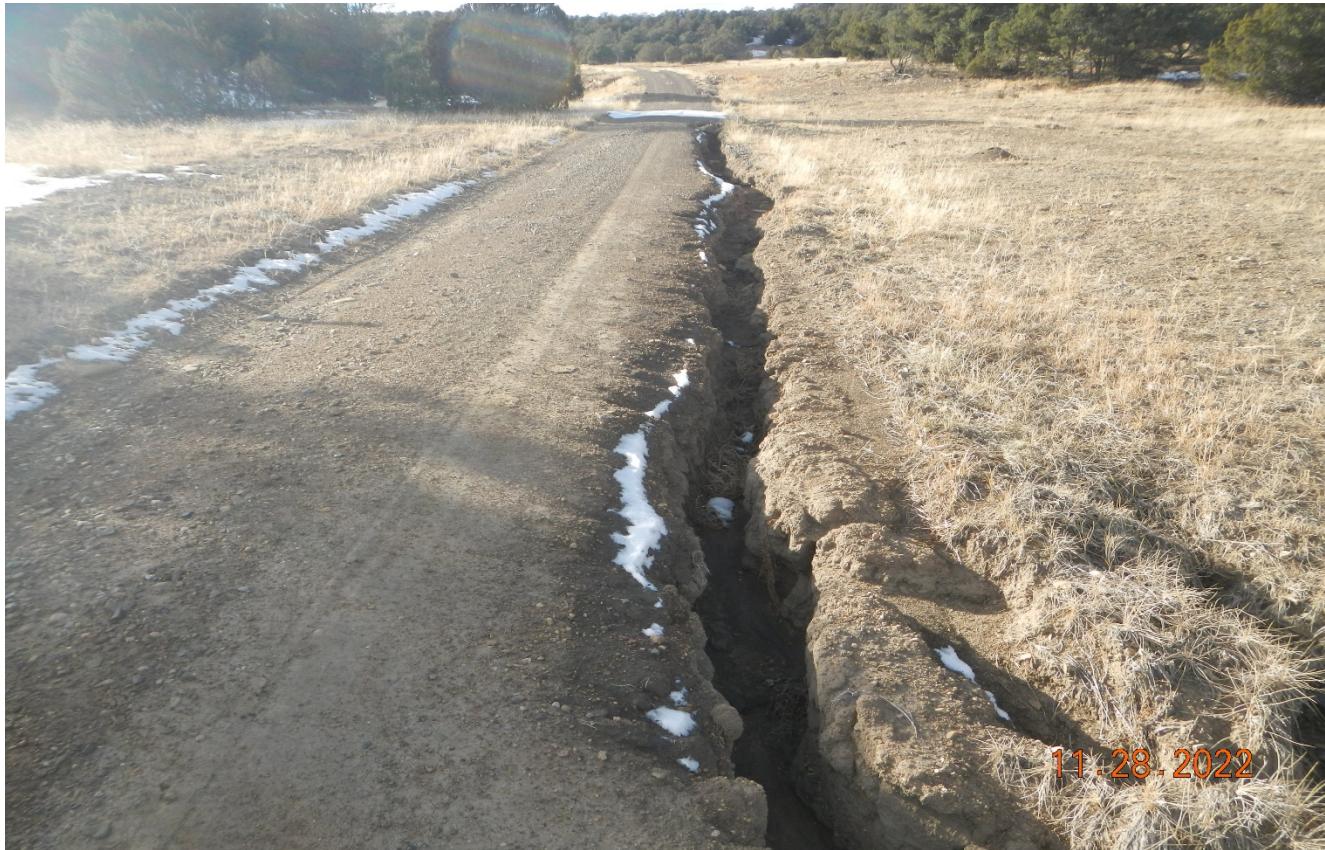
Photo 3. Along the main road at Lat/Long:37.14490,-104.67420. There is a deep erosion channel along the road that needs to be repaired.
