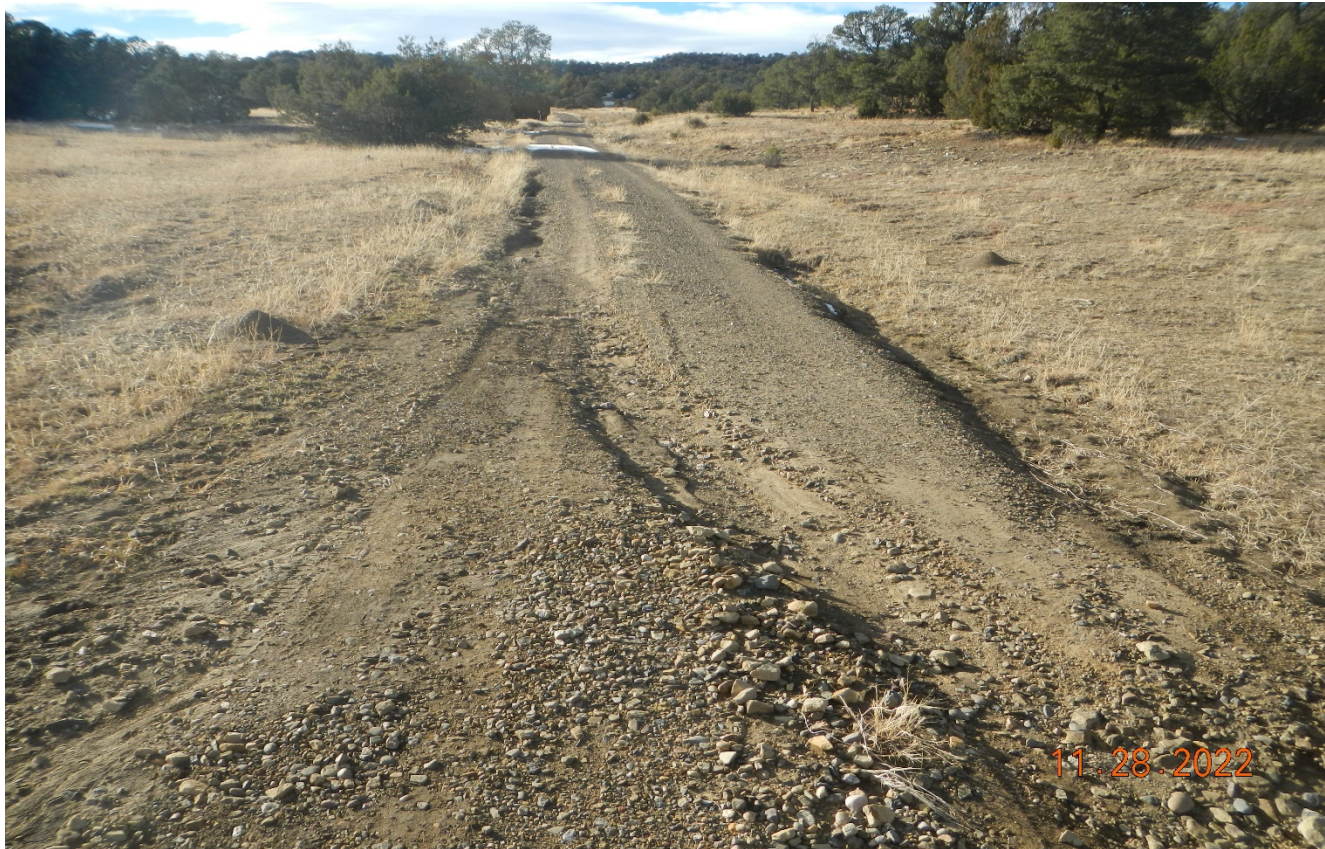
Photo 2. Along the main road at Lat/Long:37.14473,-104.67269. There is erosion along the road and stormwater is not being diverted off the road.
