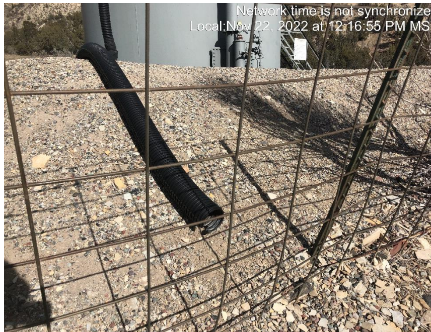
Photo #8486 Flowline heating insulation open ended.
