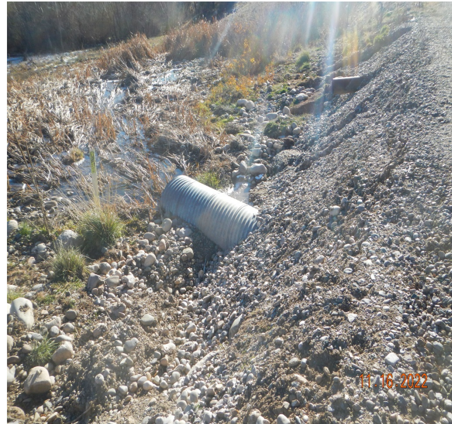
Photo 3. The culvert outlet is still partially filled in with sediment.
