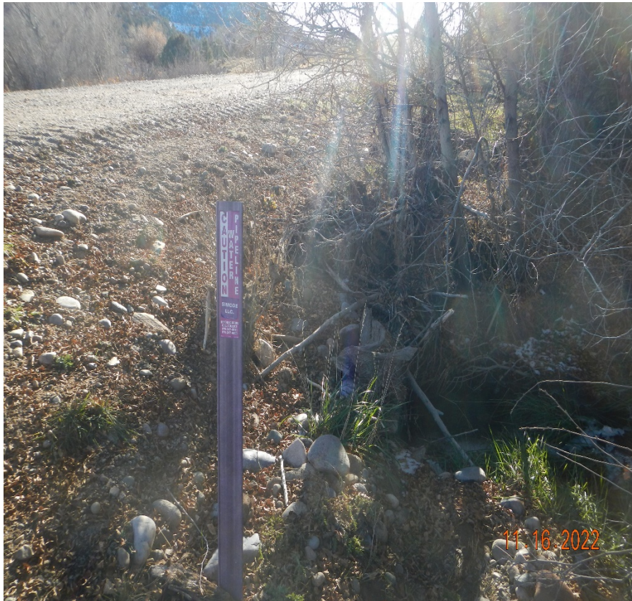
Photo 2. There is still debris at the culvert inlet that should be removed.
