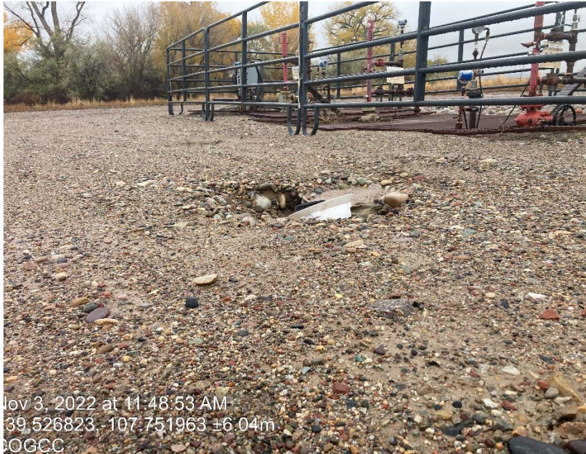
Subsidence at wells (hard hat in hole)
