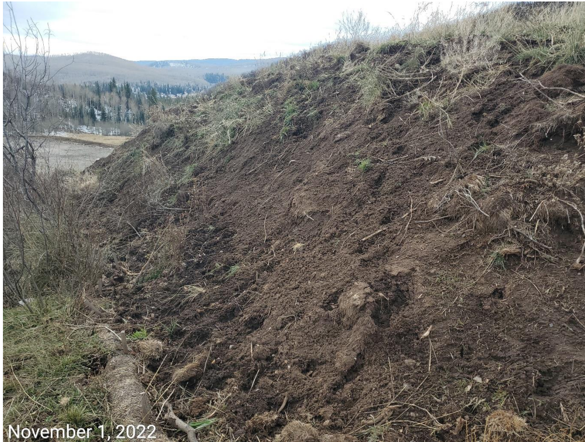
Photo 7: Continued from photo 5. Photo example showing areas of the topsoil stockpile that remains bare, and at risk to wind and water erosion; BMPs to minimize erosion, degradation and sediment transport remain missing or insufficient.
