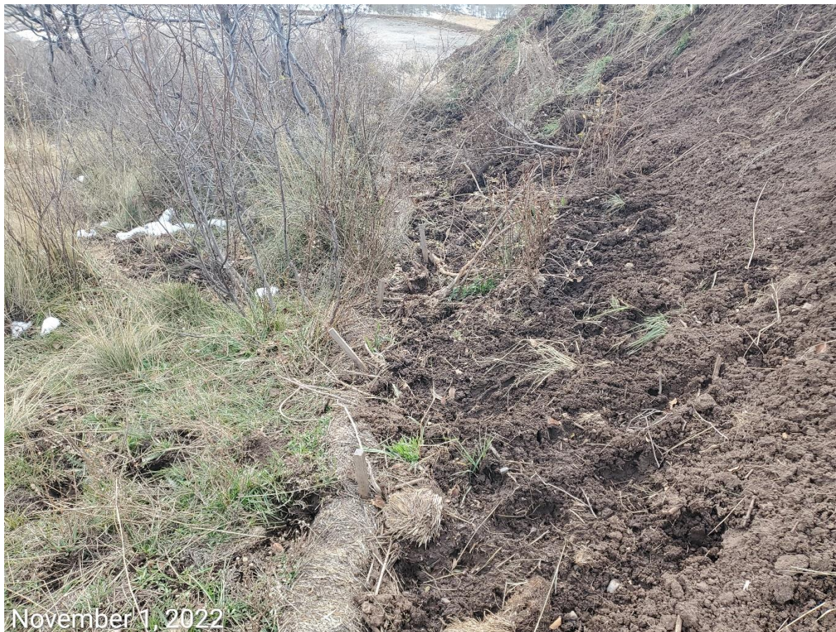
Photo 8: Photo shows Operator implemented a single row of erosion log (straw wattle) along the eastern, northern and southern perimeter of the topsoil stockpile (perimeter BMPs along the southern perimeter remains missing, see photo 5). Photo shows erosion log is not in proper functioning condition; BMP partially buried by sediment along areas of the stockpile, or flattened.
