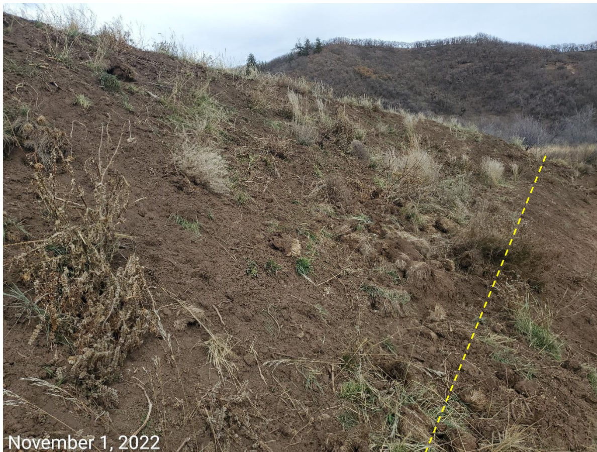
Photo 5: Photo taken from the topsoil stockpile on the north end of the Location. Photo shows large areas of the soil stockpile with bare soil at risk to wind and water erosion; control measures to minimize erosion, degradation at the stockpile, and BMPs to manage runoff and minimize sediment transport along the perimeter of the soil stockpile remain missing or insufficient. Yellow line represents top of the cut slope/base of the stockpile.
