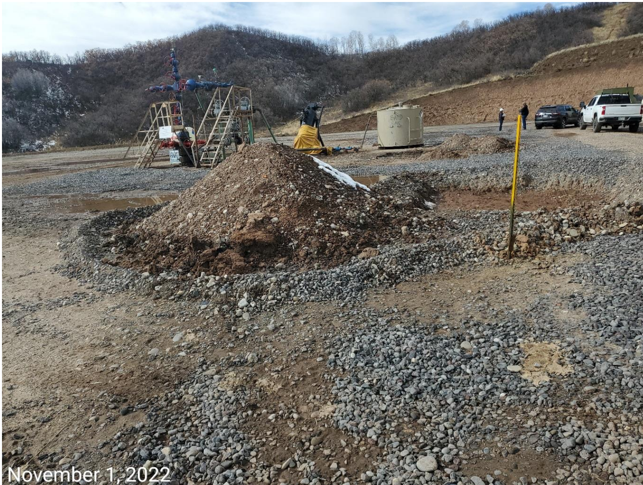
Photo 9: Photo example showing 1 of 4 stockpiles observed where Operator has conducted excavation operations to collect soil samples (see remediation proj. #23148). BMPs to protect the stockpiled soils, and to minimize erosion and sediment transport from the potentially impacted soil stockpiles are missing or insufficient. Stockpile shown in photo an example where Operator installed a berm at its base- Berms observed are unconsolidated, permeable, and have not been installed per good engineering practices
