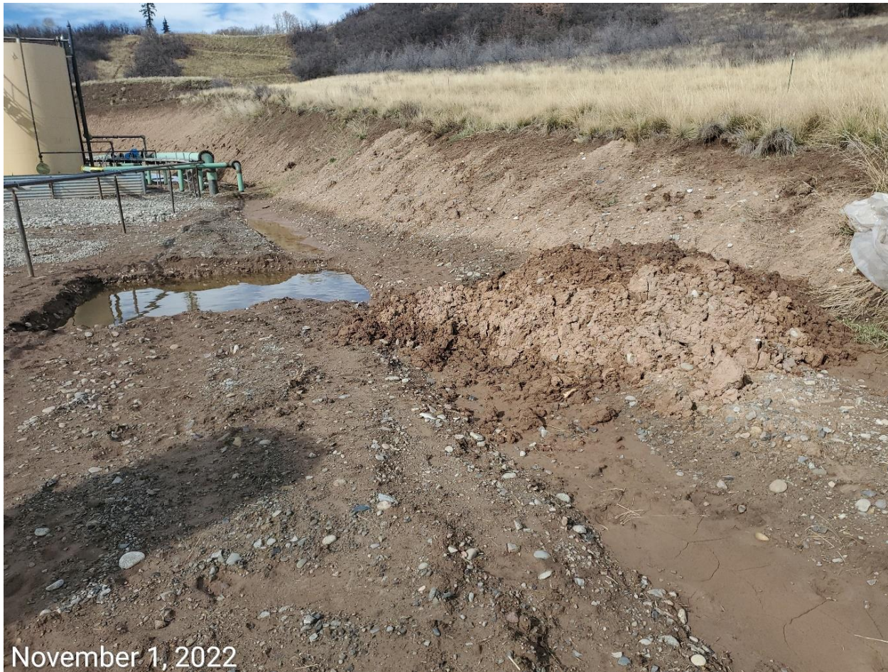
Photo 10: Photo example showing 1 of 4 stockpiles observed where Operator has conducted excavation operations to collect soil samples (see remediation proj. #23148). Photo example showing 1 of the 2 areas where Operator excavated, and placed potentially impacted soils within the perimeter stormwater diversion ditch along the east end of the working pad. In addition to missing BMPs to prevent sediment transport from the soil stockpiles, BMPs to prevent stormwater runoff from entering, or discharging from the sample pits within the ditch are also missing or insufficient, potentially increasing the risk of stormwater contamination, and contaminated discharge from the Location.
