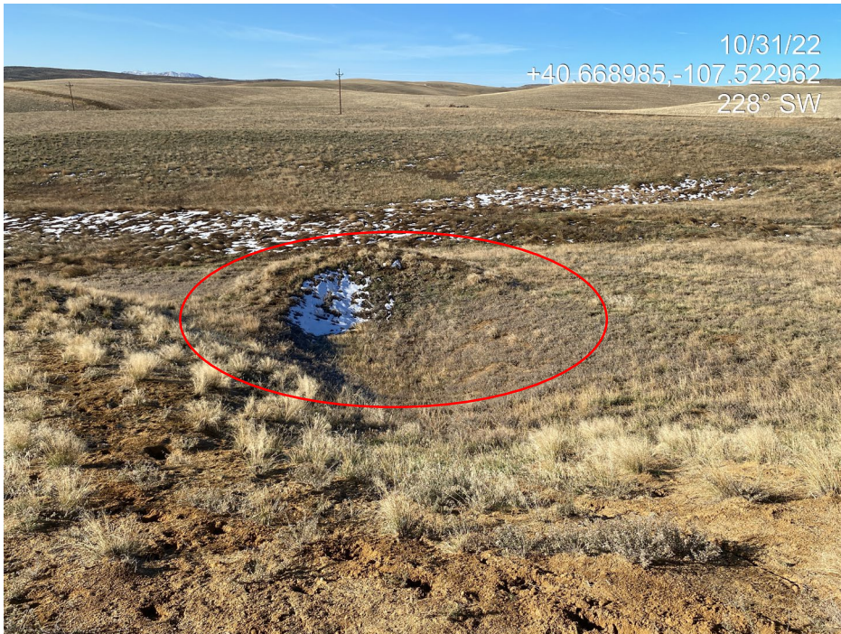
Photo 8. Photos show two pit overflow areas at the southwest of the Location. Pits have not been properly reclaimed; recontouring is required. Note natural contour of reference area; hillside gradually slopes down toward intermittent stream. Pits must be reclaimed per 1003 Rules.
