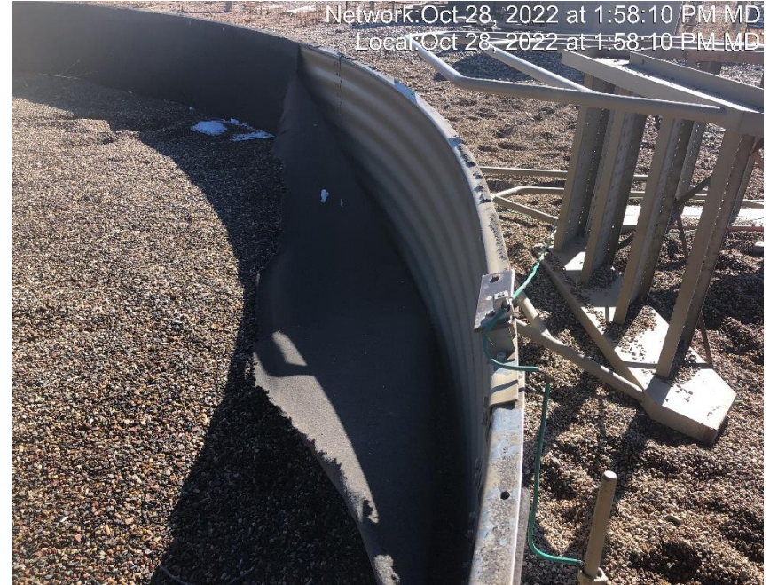
Photo #8235 Secondary containment needs repaired.
