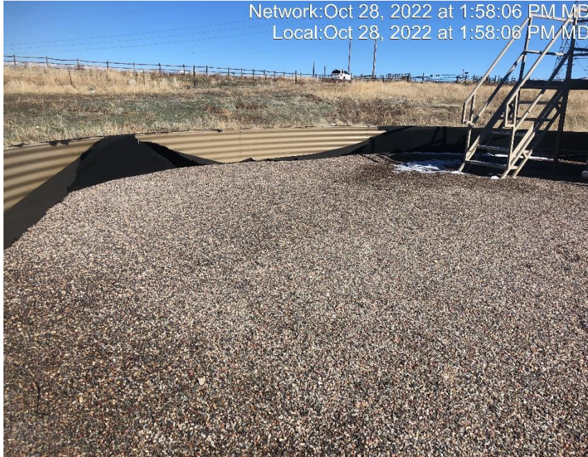
Photo #8233 Secondary containment needs repaired.
