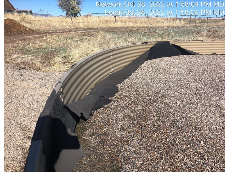
Photo #8233 Secondary containment needs repaired.
