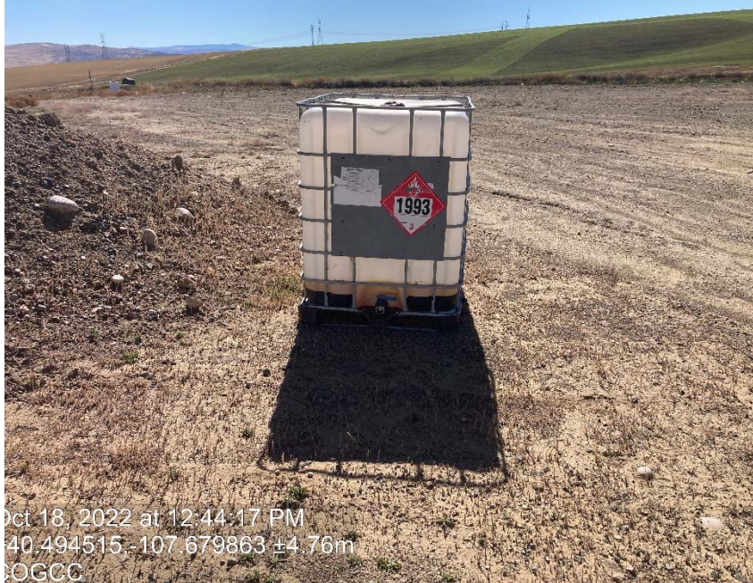
Tote not in a secondary containment
