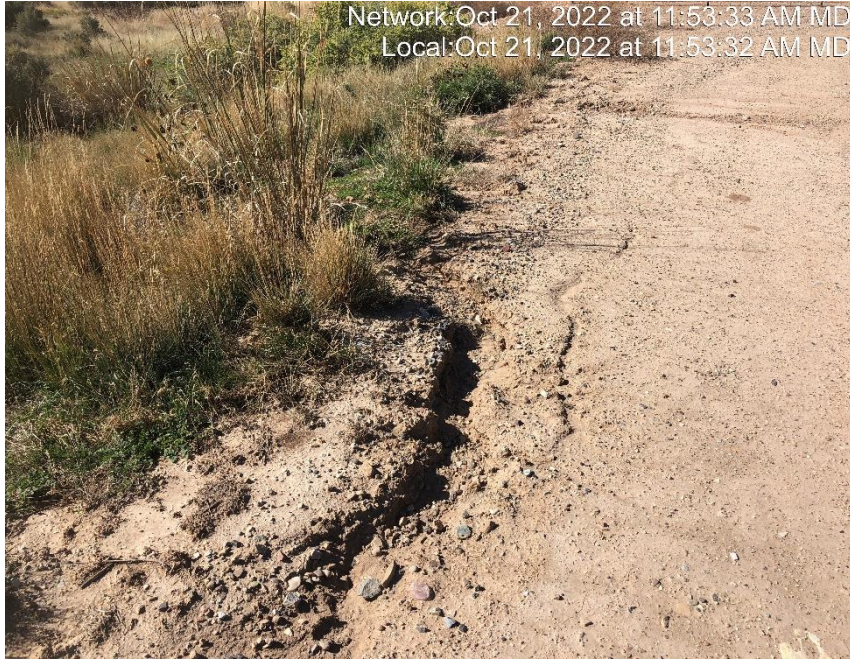
Photo #8131 Rill erosion occurring on location.
