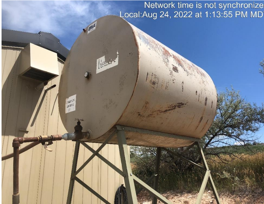
Photo #7559 Tank missing required information.
