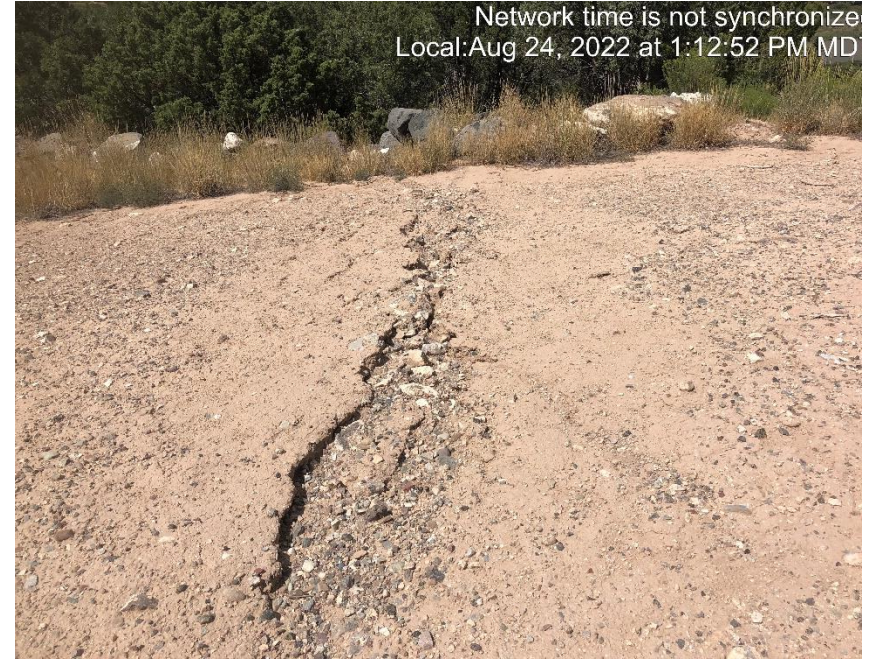
Photo #7555 Rill erosion occurring on North West side of location.
