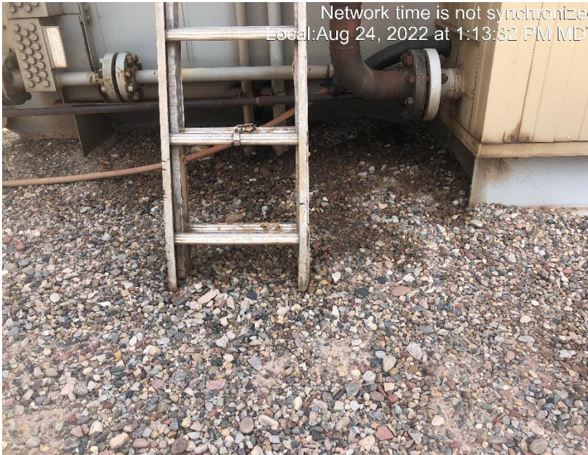
Photo #7557 Multiple places with stained soils on location.
