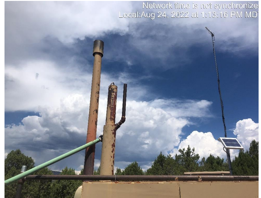
Photo #7556 Vent pipe on separator open ended.
