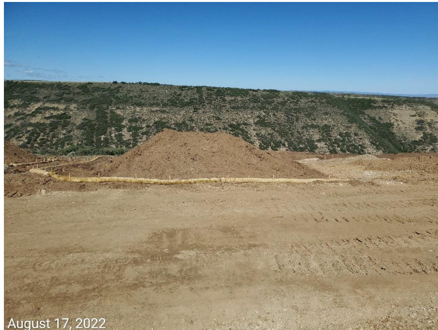
Photo 3: Photos examples of erosion logs observed at base of soil stockpiles, and along the perimeter of the Location.
