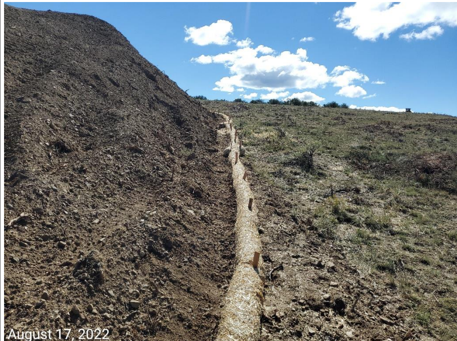
Photo 3: Photos examples of erosion logs observed at base of soil stockpiles, and along the perimeter of the Location.
