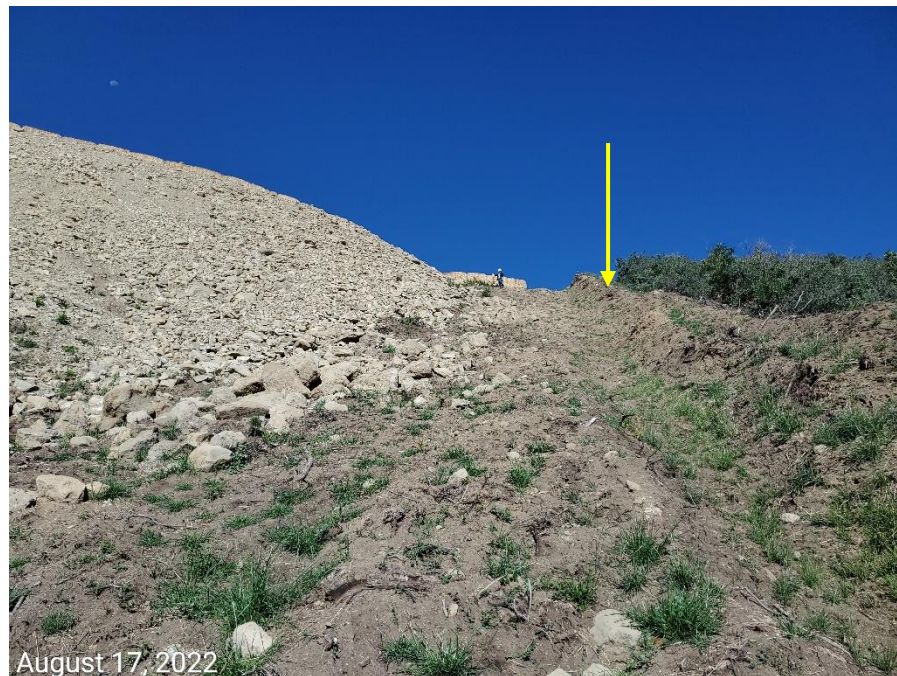
Photo 2: Photos examples showing topsoil remains in use as part of the Location's perimeter stormwater controls, specifically, one of the three sediment traps/basins on the Location, and berm.
