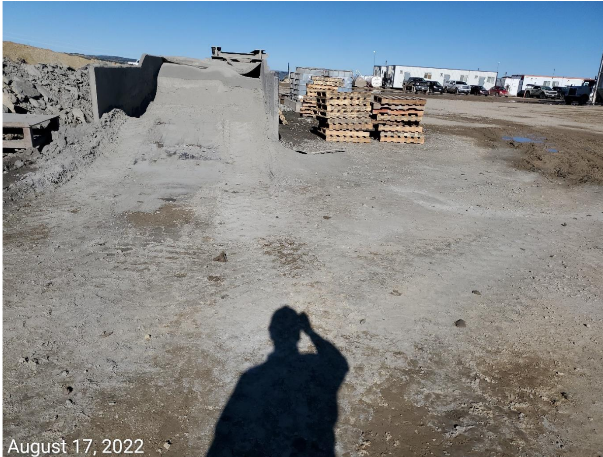
Photo 3: Previous inspection observed what appeared to be cement material spilling out of containment and upon the working pad surface. Inspection required spill to be cleaned and BMPs installed. Photo shows spill has not been cleaned. Additionally, it was observed that stormwater has come in contact with the material, and has hardened it in areas.
