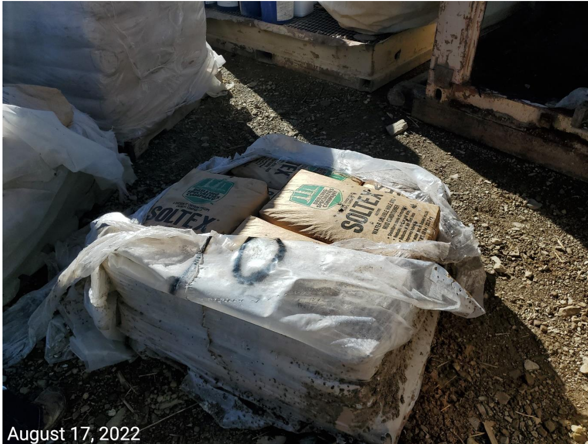
Photo 5: Photo shows improper covering BMPs resulting in precipitation/stormwater contact with materials
