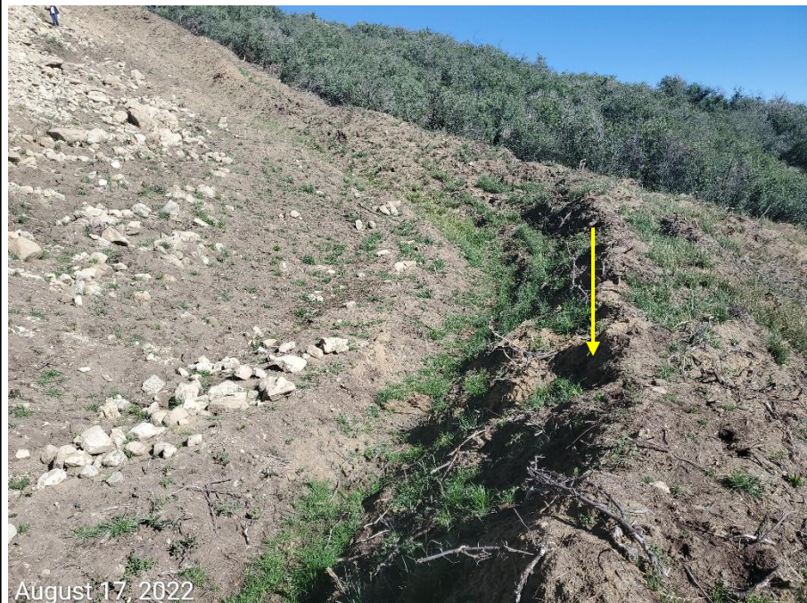
Photo 2: Photos examples showing topsoil remains in use as part of the Location's perimeter stormwater controls, specifically, one of the three sediment traps/basins on the Location, and berm.
