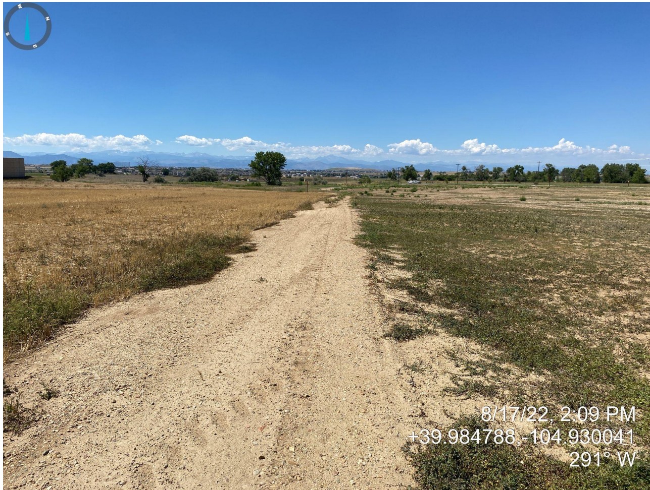
Photo 8. Access road photo taken from western portion of location/well, facing west. Photo illustrates access road has not been reclaimed, e.g. gravel/road base removed, regraded, revegetated.
