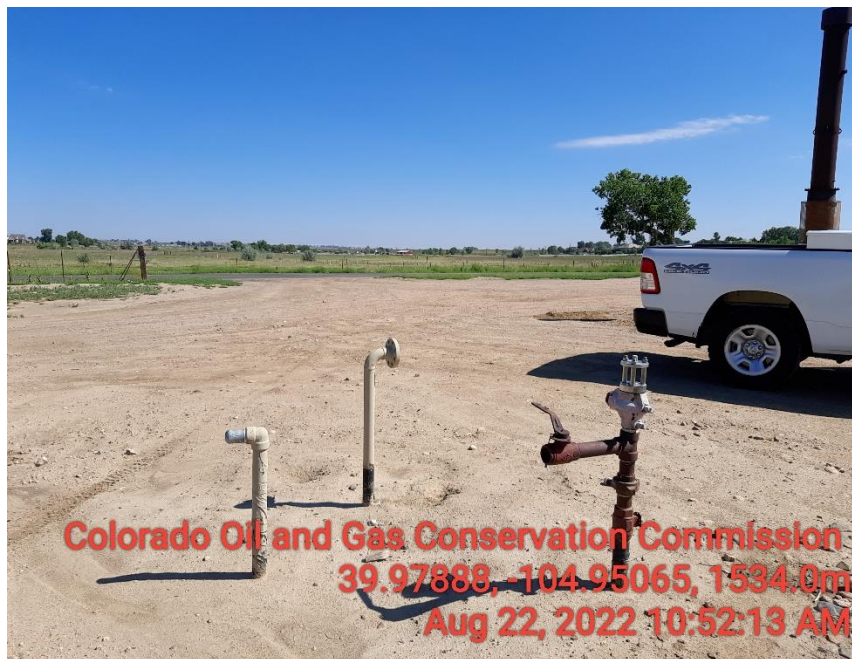
Photo 5 Meter removed lined not LOTO
