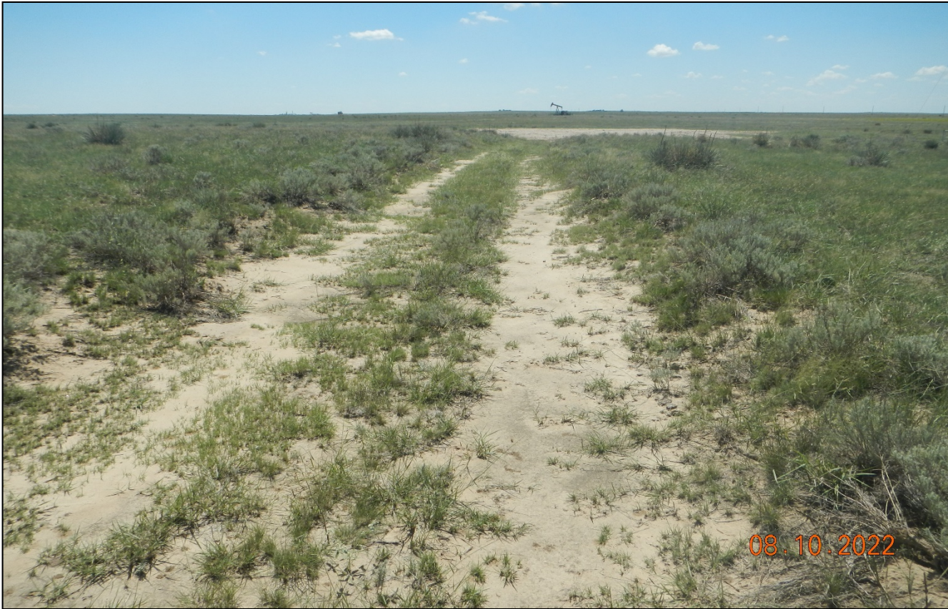
Photo 1. Facing south toward the location. The access road has not been recontoured and reclaimed.
