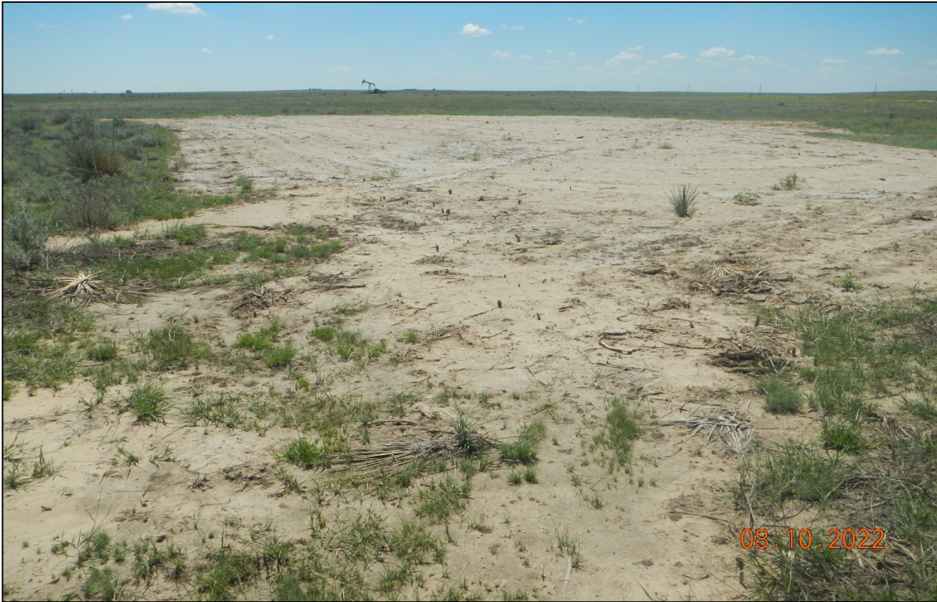
Photo 2. Facing southeast toward the location. The location has been recontoured and decompacted. Soils have not been seeded and stabilized.
