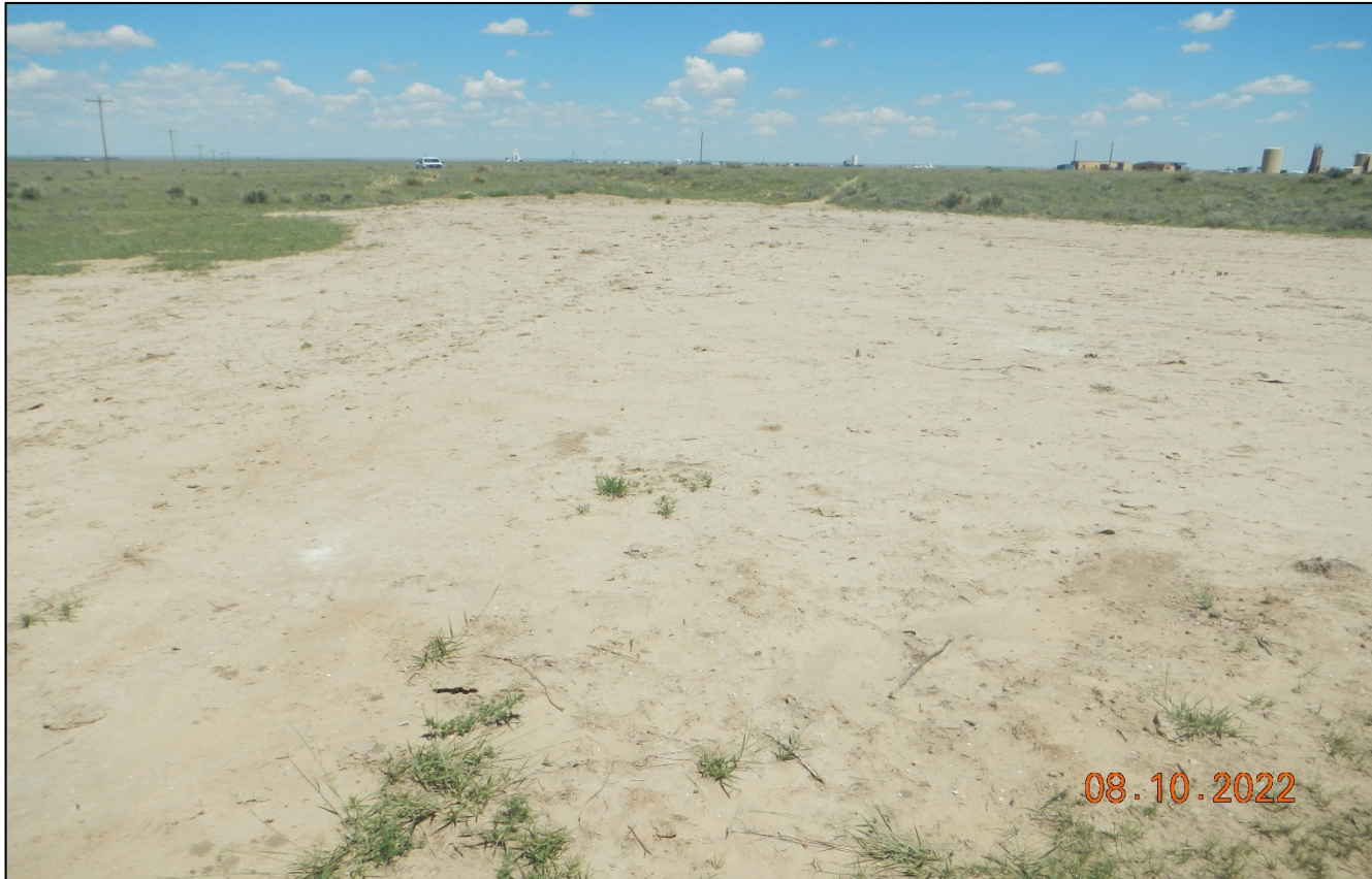
Photo 3. Facing northeast toward the location. The location has been recontoured and decompacted. Soils have not been seeded and stabilized.
