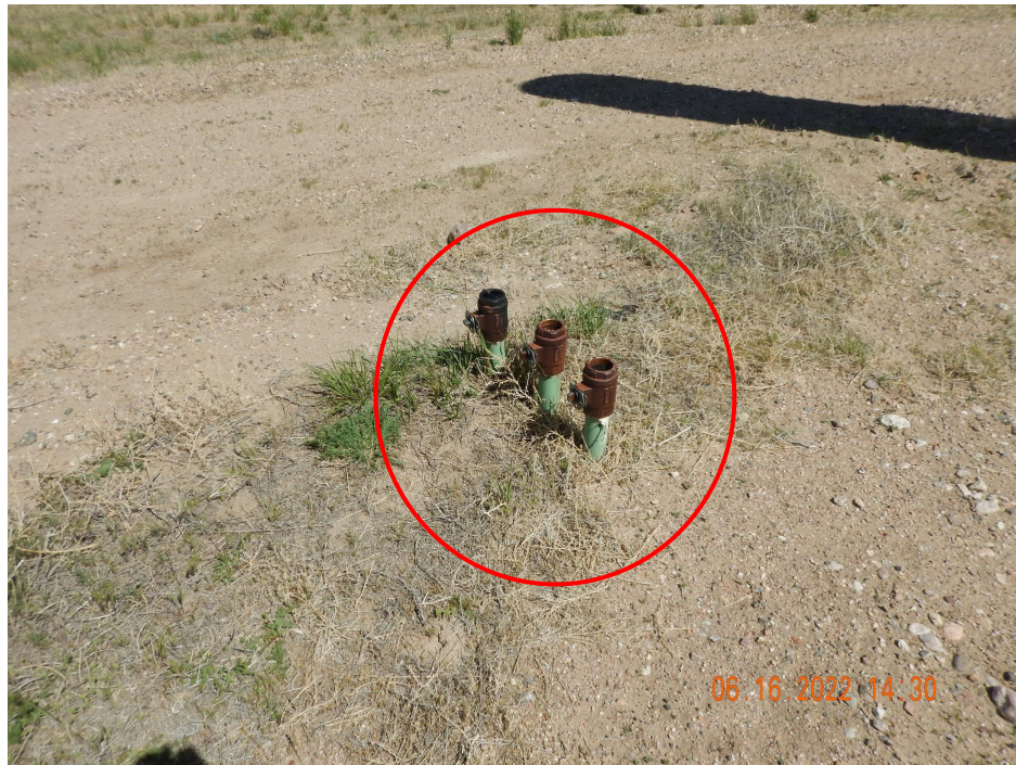
Photo 6. Photo taken from the southeastern well location, facing Southeast. Photo illustrates unused risers that are not properly abandoned per Rule 1105.
