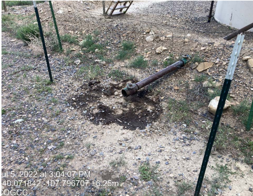
Staining/ valve lacking plug/cap
