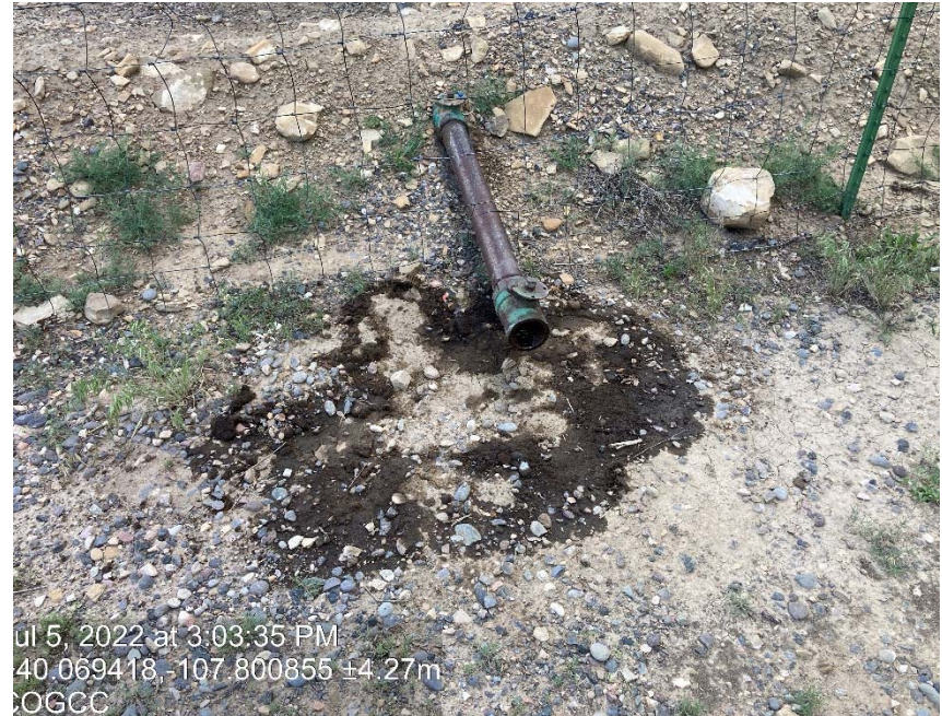
Staining/ valve lacking plug/cap
