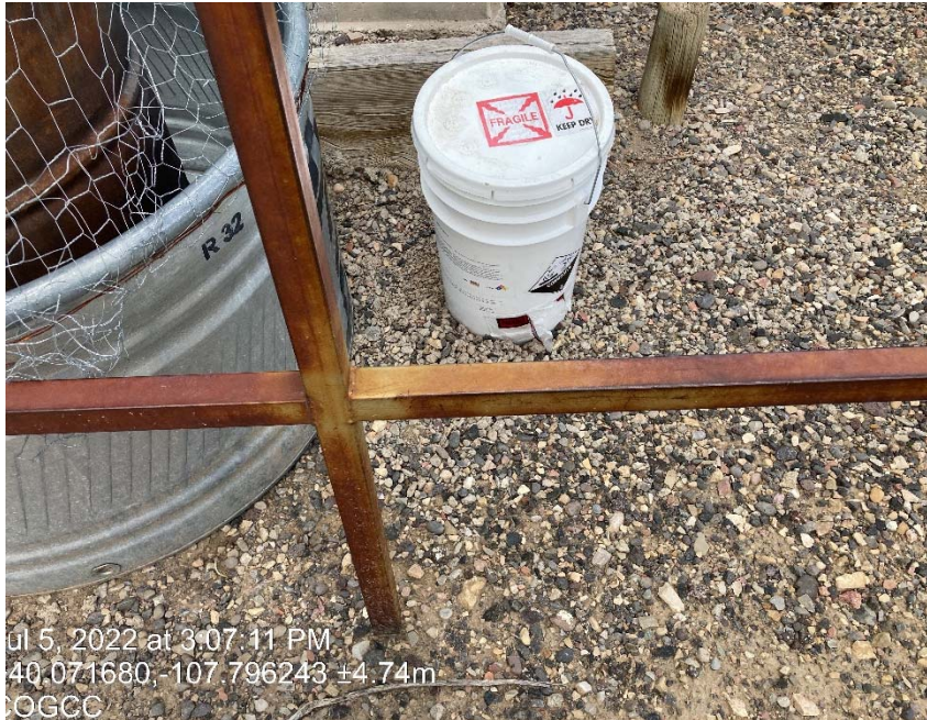
Bucket of chemicals not in a containment
