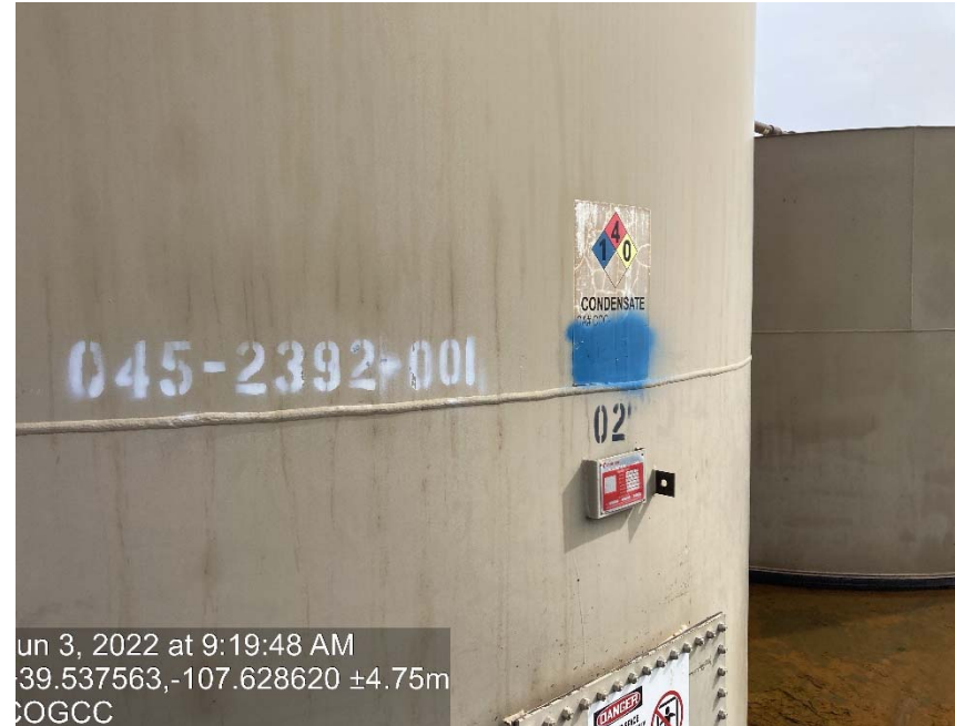
Tank missing labeling
