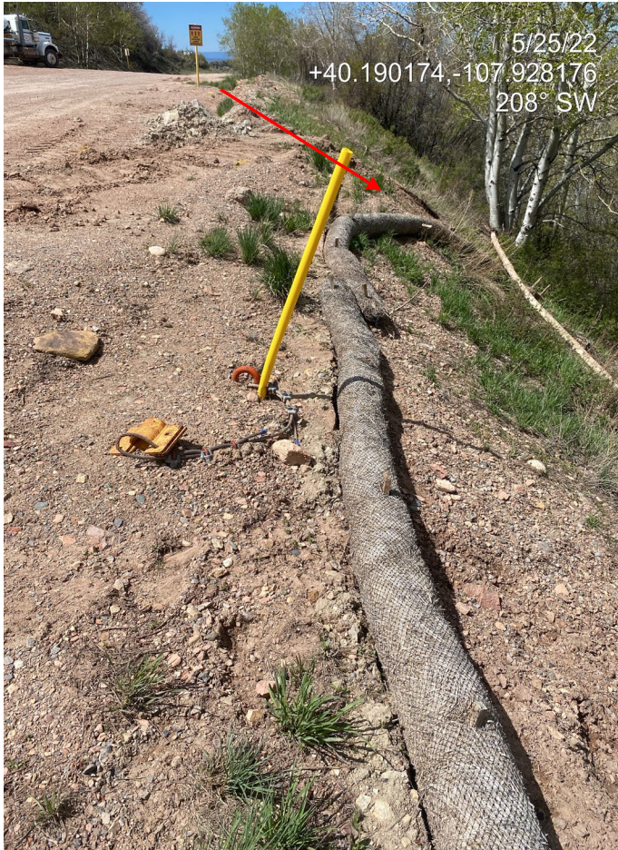
Photo 5. Photo taken from the northwest of the Location shows a straw wattle in disrepair and not functioning to control sediment transport from the Location.
