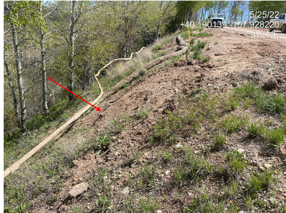
Photo 4. Photo taken from the northwest of the Location shows a straw wattle in disrepair and not functioning to control sediment transport from the Location.
