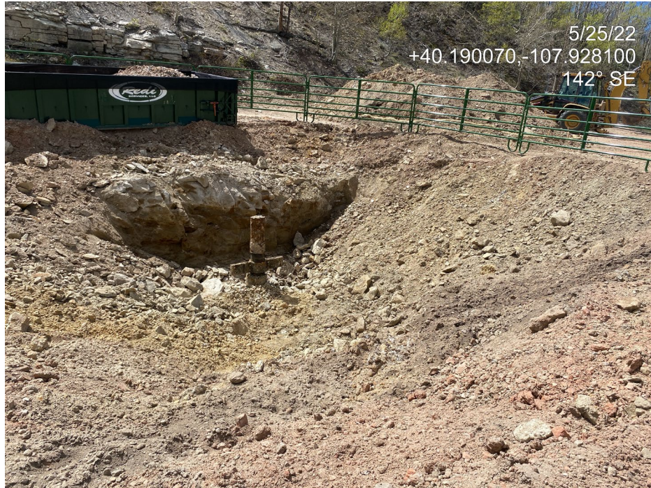
Photo 1. Photo taken from the center of the Location shows the excavation around the wellhead. Fence panels completely enclose the area and the slope of the pit is sufficiently gently to allow for wildlife egress.
