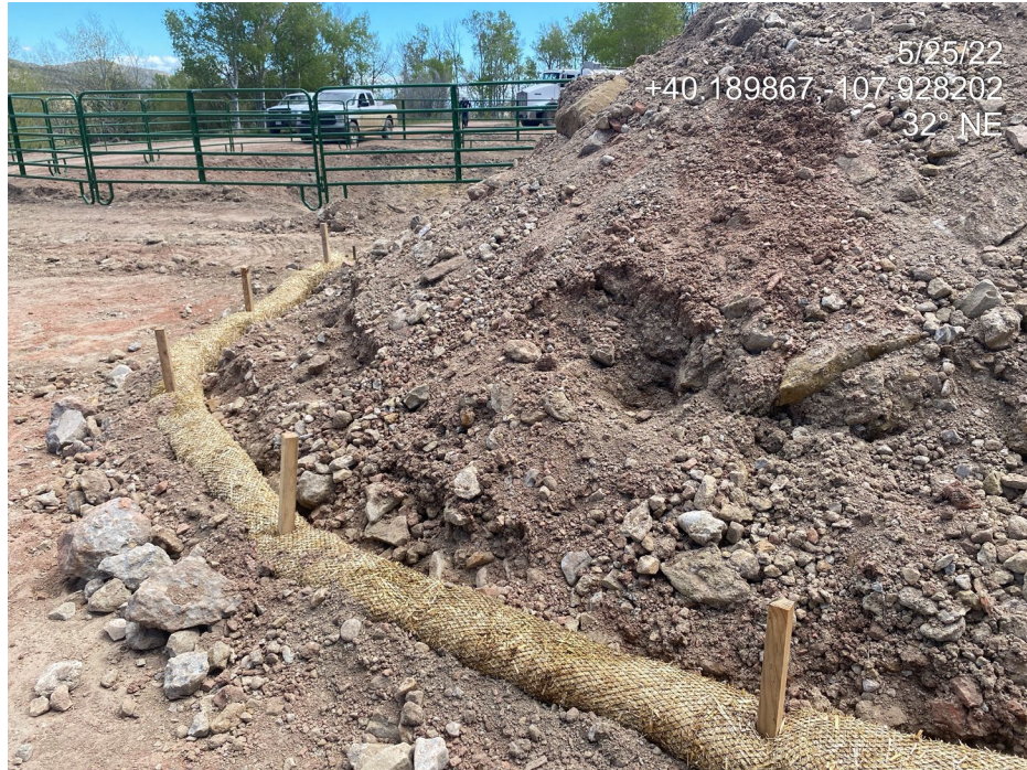
Photo 3. Photo taken from the south of the Location shows a pile of material excavated from around the well. A straw wattle has been installed as a control measure to prevent E&P waste from migrating off Location.
