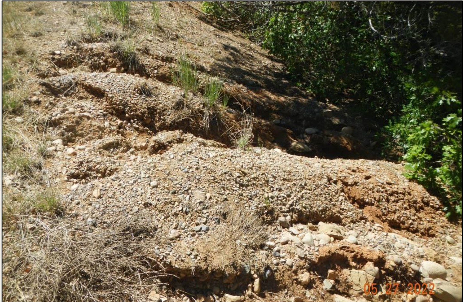
Photo 4. View of erosional channeling in the southern fill slope, approximately 1-2ft wide and deep.
