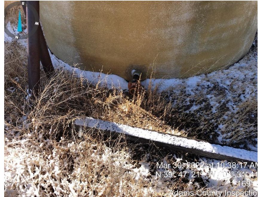
Photo #10 Debris and no bull plug in P/R water tank.
