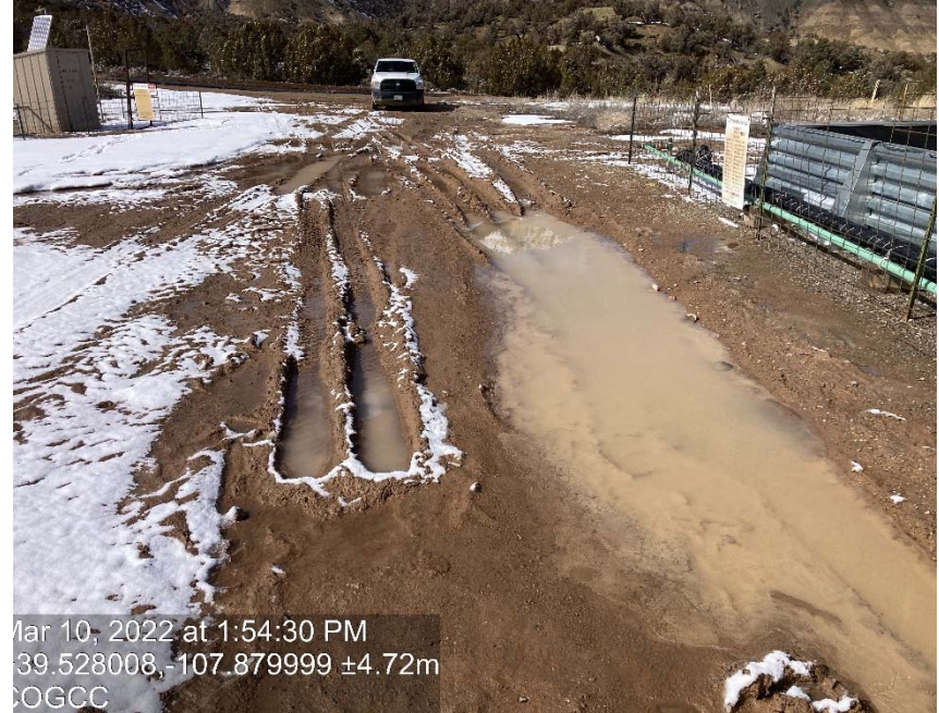
Location/ lack of stabilization-compaction
