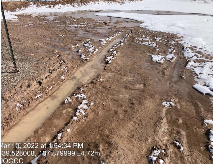
Location/ lack of stabilization-compaction
