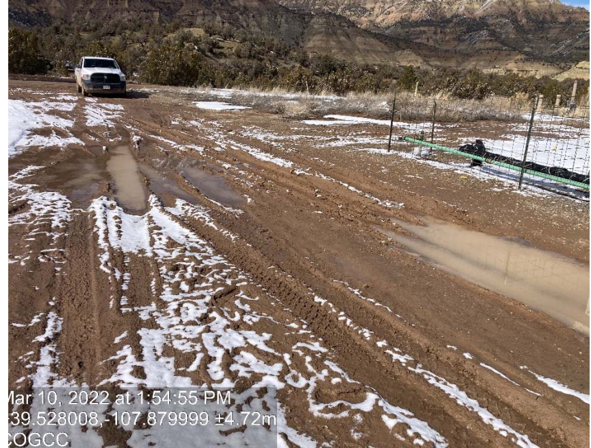
Location/ lack of stabilization-compaction
