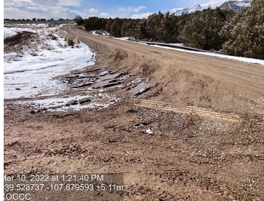
Location/ lack of stabilization-compaction
