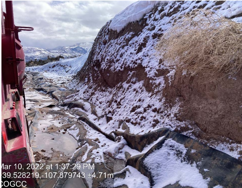
Cut slope lack of stabilization
