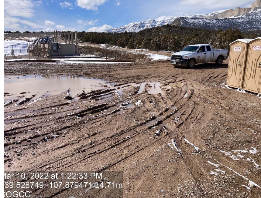
Location/ lack of stabilization-compaction
