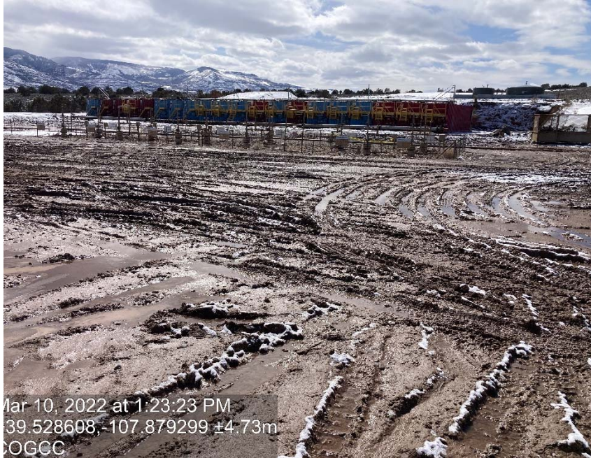
Location/ lack of stabilization-compaction
