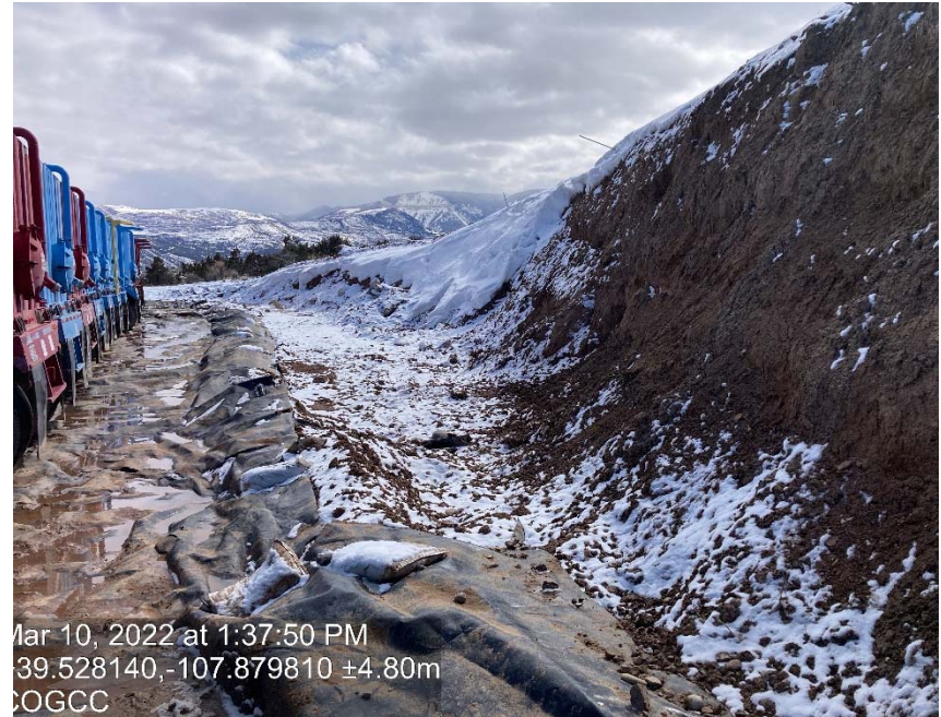
Cut slope lack of stabilization
