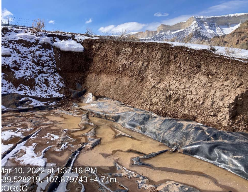
Cut slope lack of stabilization
