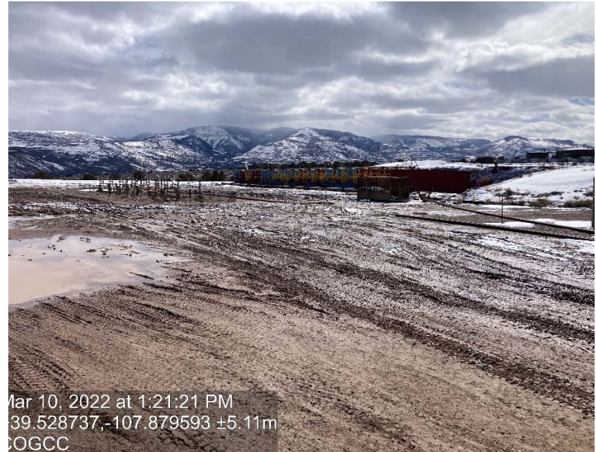
Location/ lack of stabilization-compaction
