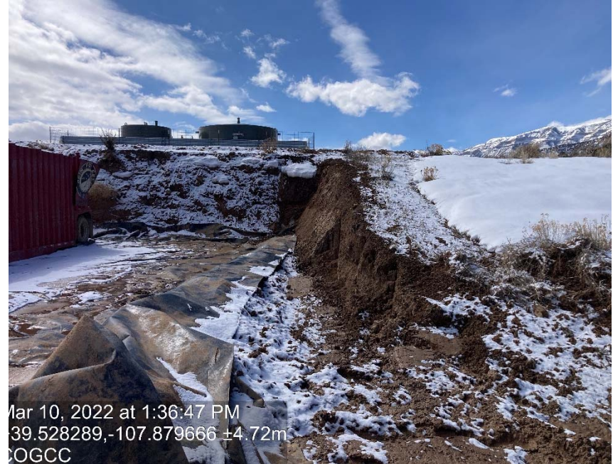
Cut slope lack of stabilization
