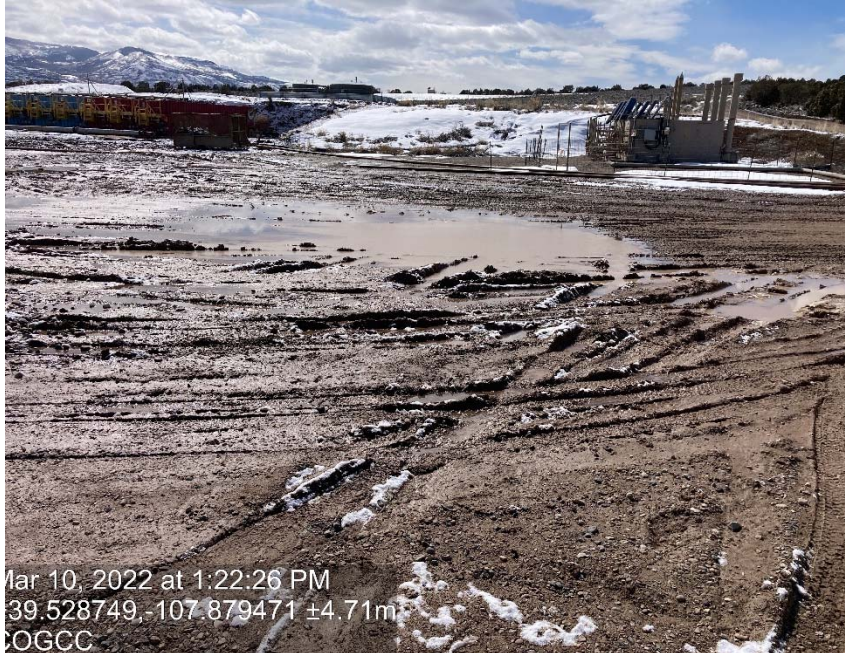
Location/ lack of stabilization-compaction
