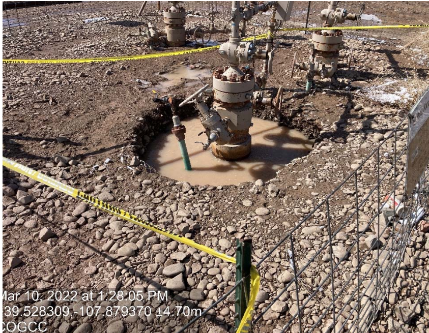
Well head leaking
