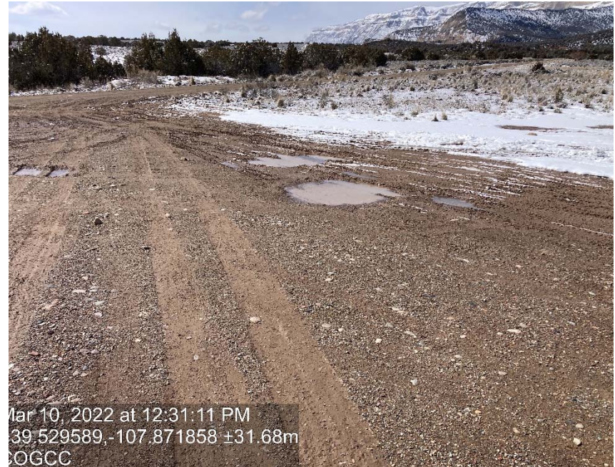
Lack of stabilization/ compaction
