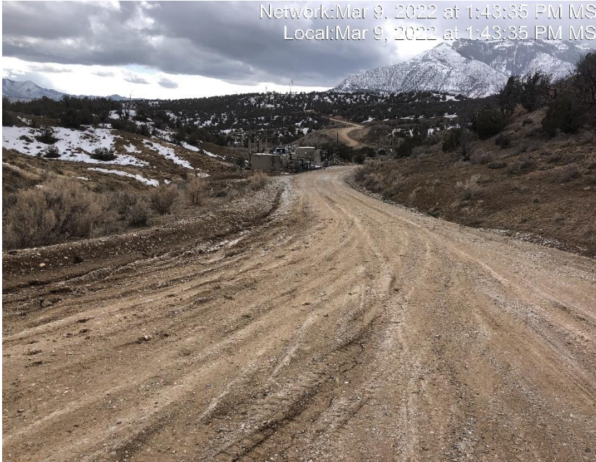
Photo #6122 Insufficient tracking control at entrance to location.
