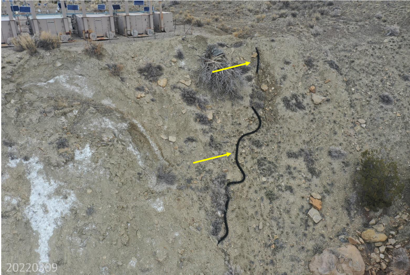
Photo 7: Photos taken with use of a sUAS. Photo shows slope drain on the south end of the Location; the slope drain has not been installed in accordance with good engineering practices, and is not in proper functioning condition; drain pipe has been cut halfway down slope; remaining pipe not in use is considered debris and requires removal. Slope drain has not been properly secured or constructed with an engineered outlet, which has resulted in stormwater degradation at the outlet. Stormwater and erosion control measures to allow for proper stormwater discharge, and to minimize off site degradation is missing or insufficient.
