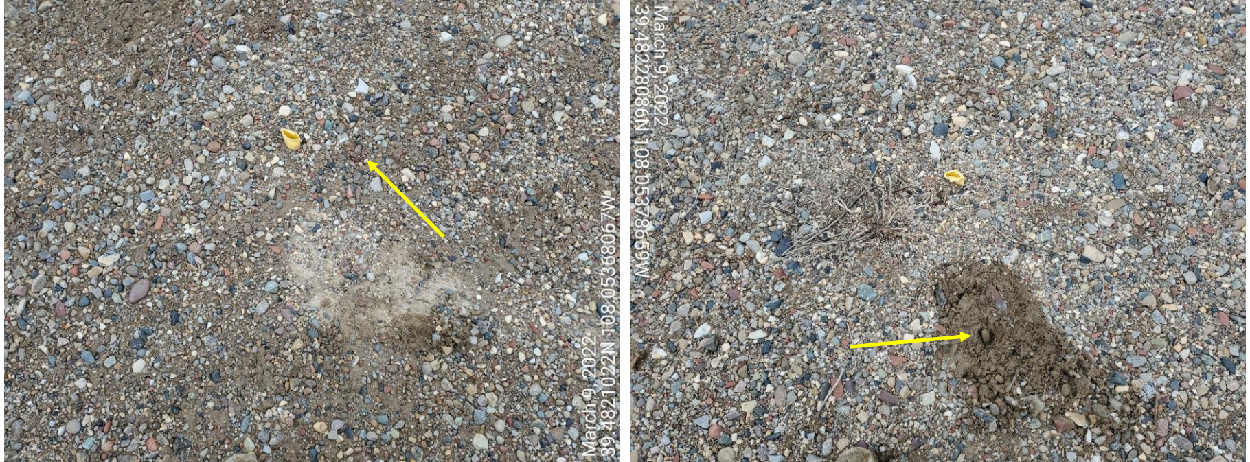
Photo 10: Photos taken from the working pad of the Location. Photos provide examples showing control measures to stabilize the working pad, minimize rutting, tracking and sediment transport remains missing or insufficient.
