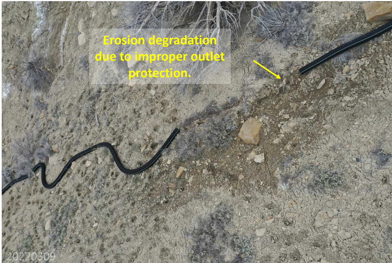
Photo 8: Continued from photo 7. Photo shows slope drain pipe has been cut halfway down slope. Photo also shows slope drain has not been properly secured or constructed with an engineered outlet (per good engineering practices), which has resulted in stormwater degradation at the outlet. Stormwater and erosion control measures to allow for proper stormwater discharge, and to minimize off site degradation is missing or insufficient.
