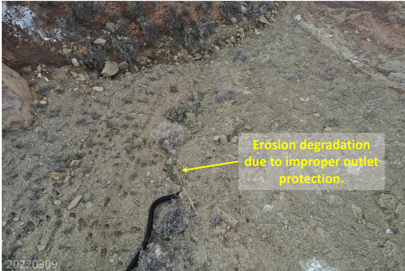
Photo 9: Continued from photo 8. Photo shows the outlet of the lower section of slope drain pipe that has been cut off; this section of pipe is now debris. Photo shows that a properly engineered outlet was also not constructed at this outlet, resulting in erosion degradation when this section of pipe was still in use. Stormwater and erosion control measures to allow for proper stormwater discharge, and to minimize off site degradation is missing or insufficient.
