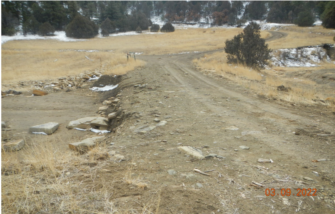
Photo 1. Facing southwest along the main road in Martinez Canyon. Last years flood caused stormwater to flow across the road due to culverts plugged up with debris.
