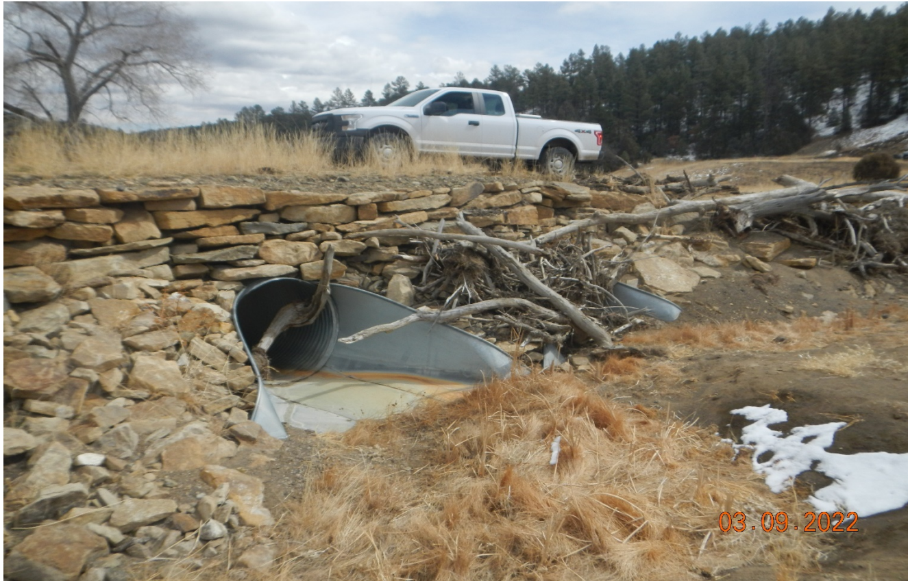
Photo 2. The culverts along the canyon crossing are filled in with debris which needs to be removed.
