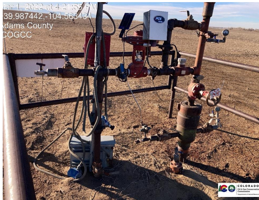
Pic 1 Flowline valves, and master valve were in the open position at time of inspection. Valves were put in close position, and LOTO installed on master valve. All P3 wells are in need of annual bradenhead test.
