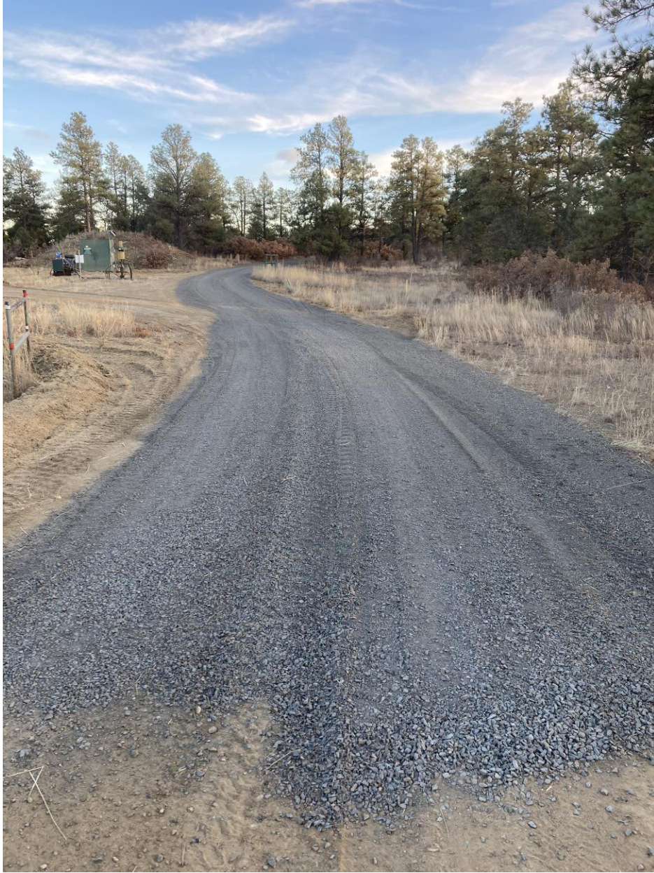
Road base has been added for stabilization
