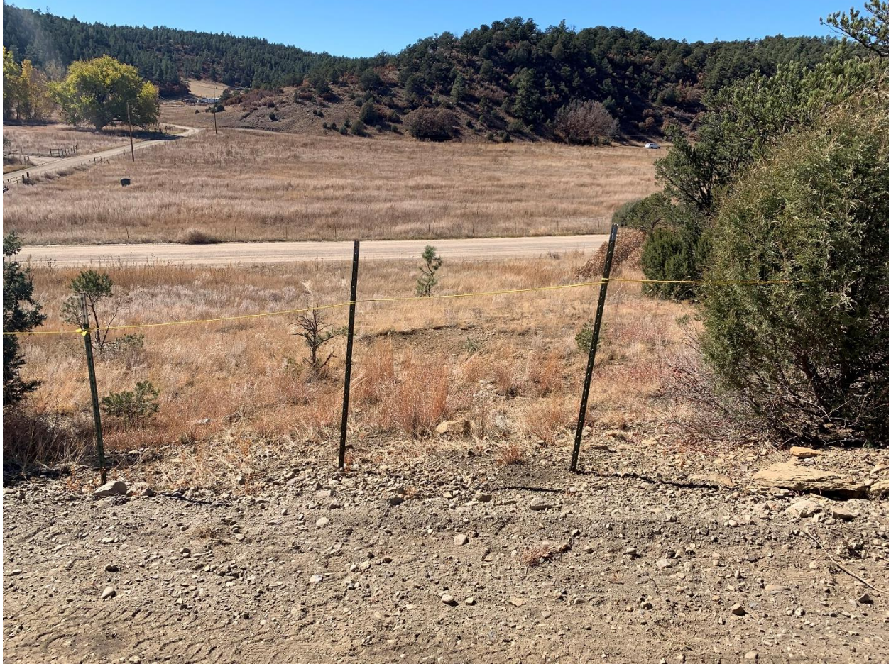
Fixed vehicle tracks raked and repaired; all oil and gas vehicle will stay inside within access road to comply with Rule 1002.e.
