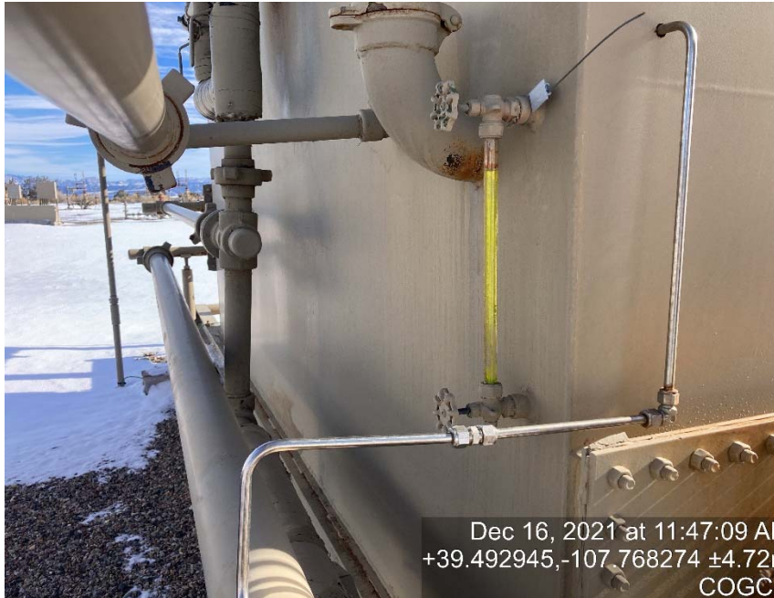
Sight glass on storage tank shows fluid in tank Storage tank lacking labeling
