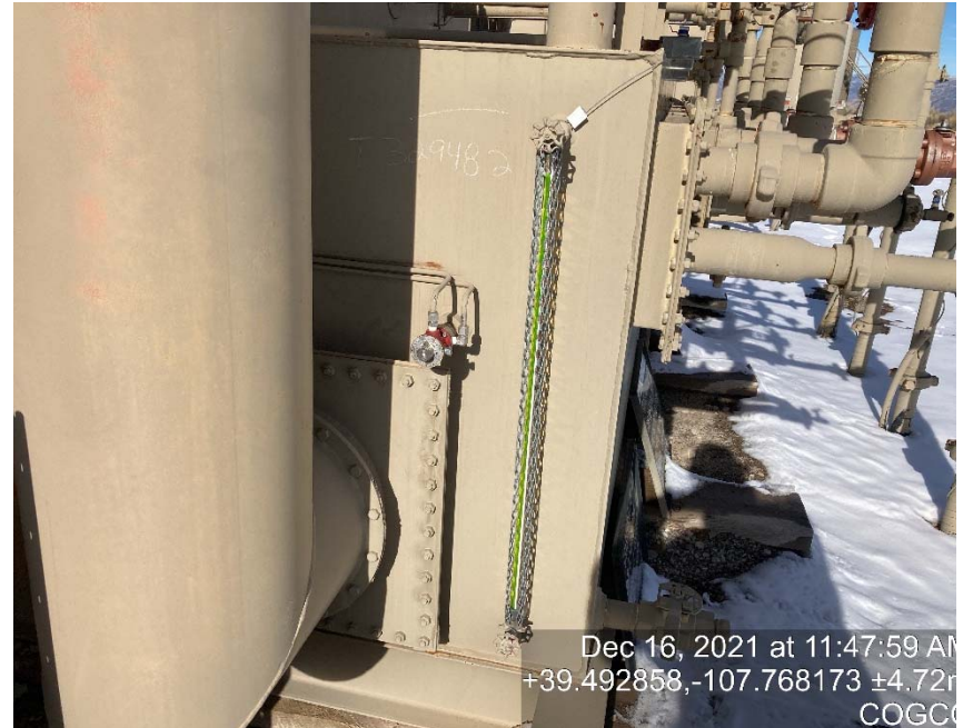
Sight glass on storage tank shows fluid in tank Storage tank lacking labeling
