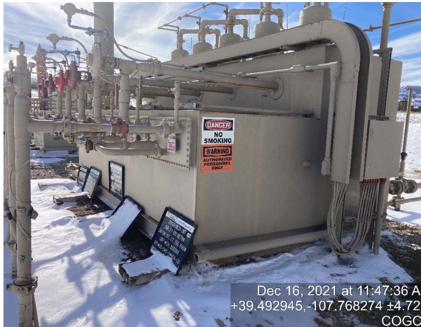
Storage tank lacking labeling
