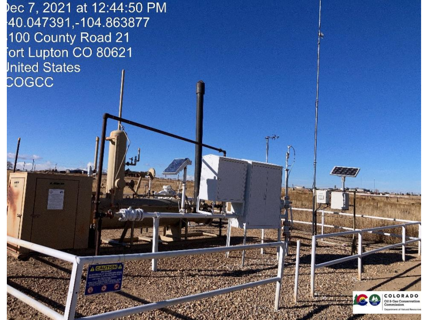
Pic 4 Separator, gas meter run, Pig Station, Automation communication equipment.
